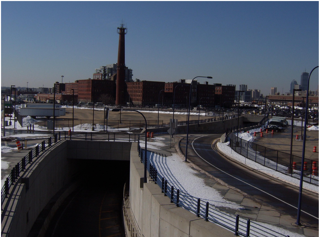
Exit Tunnels beneath the Fort Point Channel Historic District, 2006.
