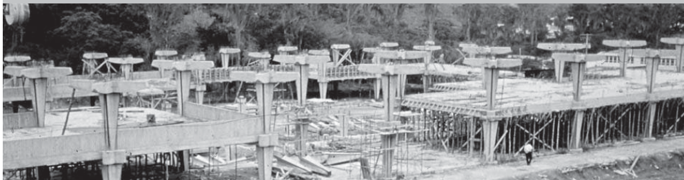
↑ With the upper story columns in place, the next level is ready to be formed and concreted.
