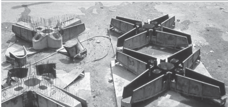
↑ With the upper story columns in place, the next level is ready to be formed and concreted.
