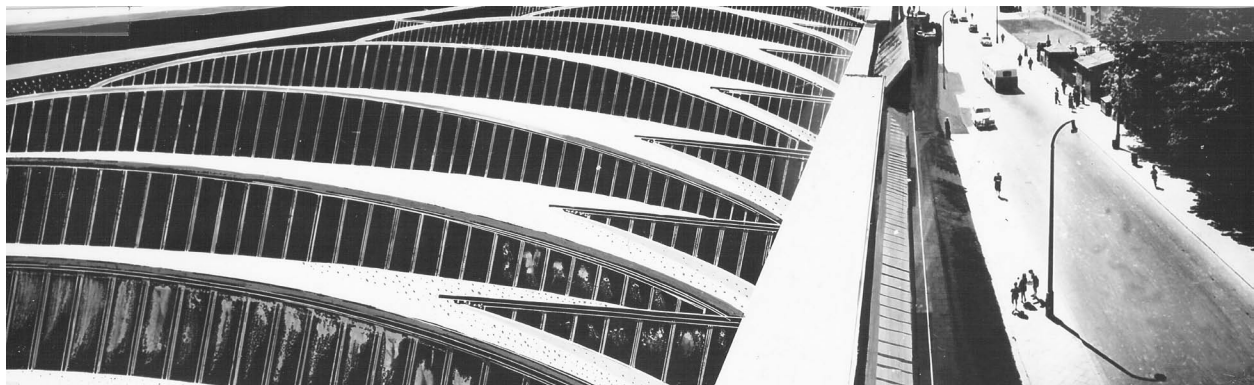
Optimal long-span thin shell concrete roofs for factories, Warsaw c.1960 [Zalewski 2006]
