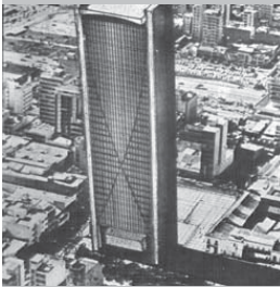
↑ This structure would use even less material if the funicular braces ran to the ground.
