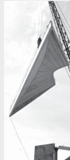
↑ Each vault is made up of four identical precast segments.
