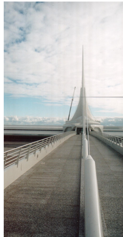
Milwaukee Art Museum, pedestrian bridge with view to central hall with brise-soleil under construction, 2001
