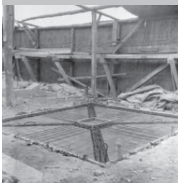
↑ Each floorplate component had internal reinforcing bars.
