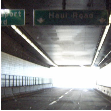
Existing view of exit ramp with abundant glare
