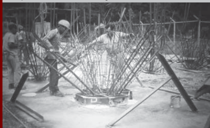
↑ Workers assemble reinforcing for the structural elements.
