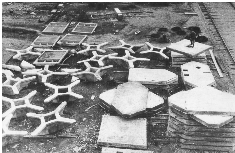
Concrete components for capital system ready for assembly, Warsaw, Poland [Zalewski 2006]
