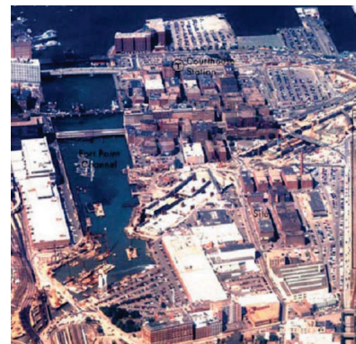
The entire site dug up 40 to 50 feet down during tunnel construction in the late 1990s [BRA 2005]
