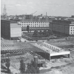
An aerial construction view shows the site within central Warsaw.
