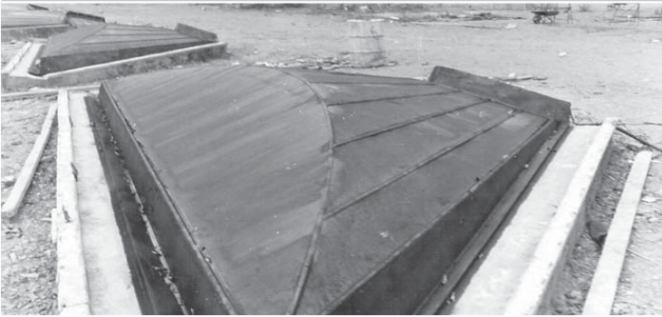
⬇ The formwork for the roof vault segments includes pipes through which water is pumped to separate the concrete from the form. These produce a ribbed pattern on the interior of the shells.
