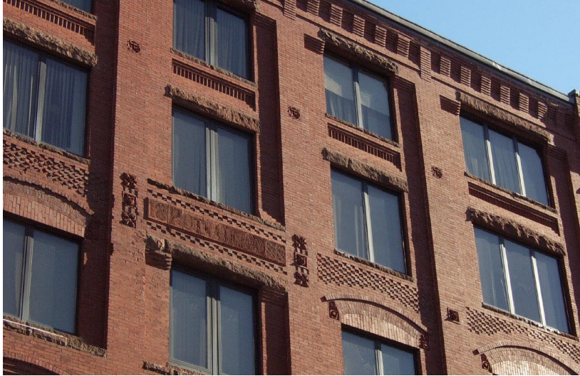
Panel Brick Detailing, 2006
