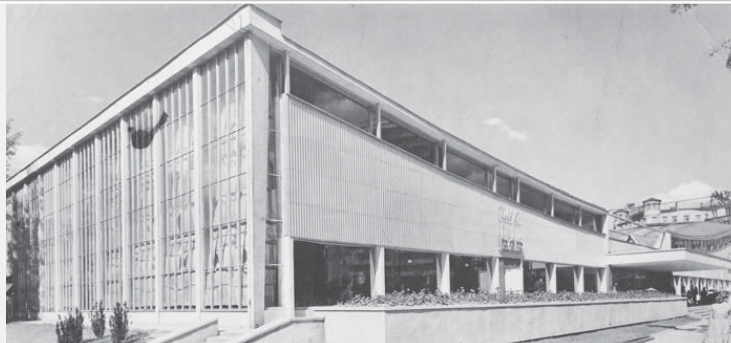
↓ The roof terminates with a cable rather than an arch at each side for a more unified appearance.
