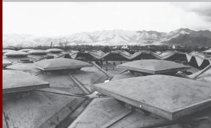
↑ A canopy shelters each oculus but allows free convective airflow.
