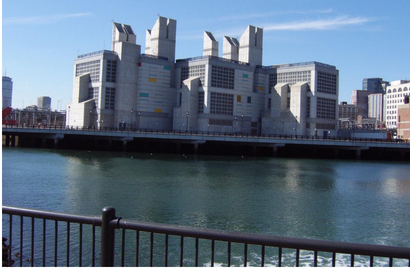
Vent Building over Big Dig tunnels, adjacent to Fort Point Channel, 2006
