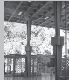
↑ The lower lobby features truncated columns that support full columns for the floor above.
