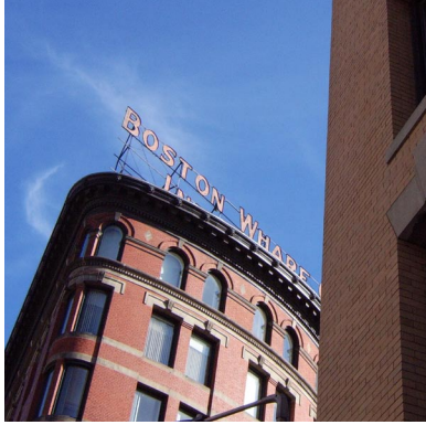
Historic buildings at the rounded corner of Melcher and Summer Streets, 2006
