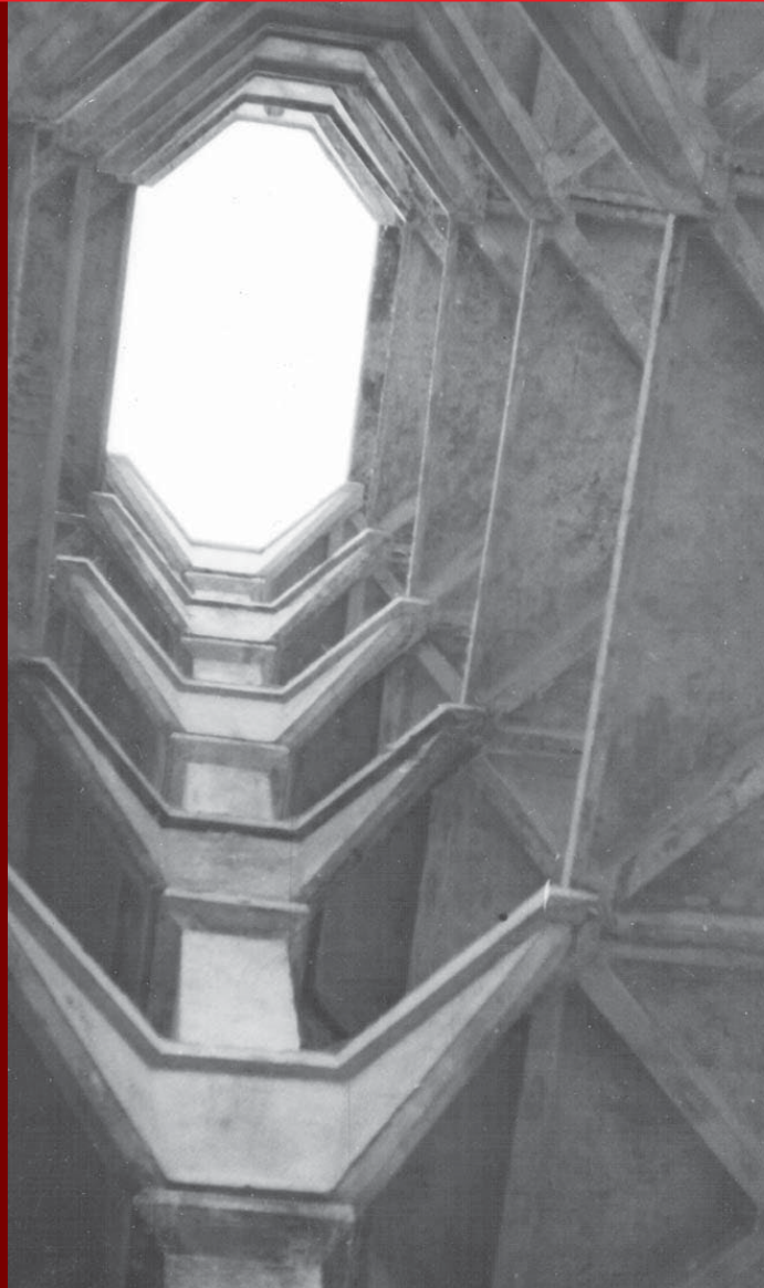
↑ Omitting hexagonal panels allows for multistory utility shafts.
