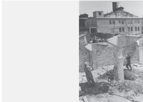
↓ Precast elements were guided down onto columns within the constrained site context.
