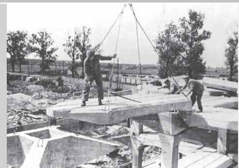
↓ The construction process required allowances for tolerances and assembly; the post-tensioning cables under the final pour of the concrete slab for the finished floor made the system monolithic and filled tolerance gaps.
