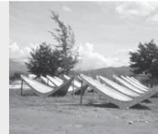
↓ The precast roof vault elements are as thin as 4 cm. (1.6 inches) in places.
