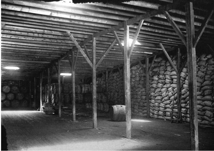
Timber loft interior c. 1900 [Quin 2001]
