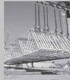
↑ The trusses were lifted in their folded position.
