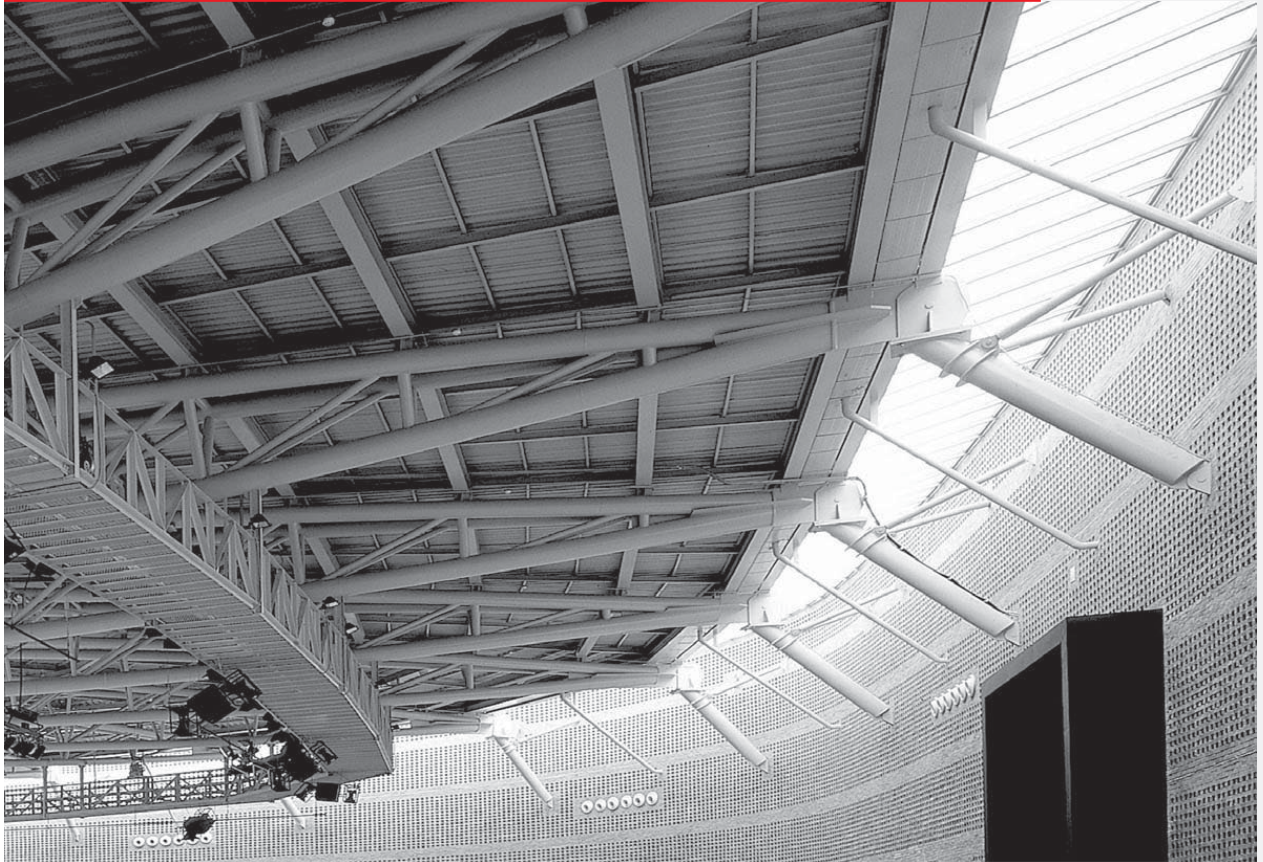
↑ The large inclined tubes carry the weight of the roof to the walls; two smaller tubes brace each large tube laterally. The tubes midway between the large tubes are for roof drainage.
