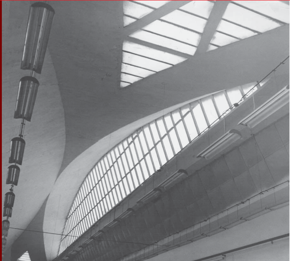
↑ All the shells feature generous daylighting by means of large clerestory windows.
