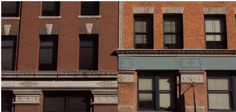
Facade juncture along Summer Street, 2006
