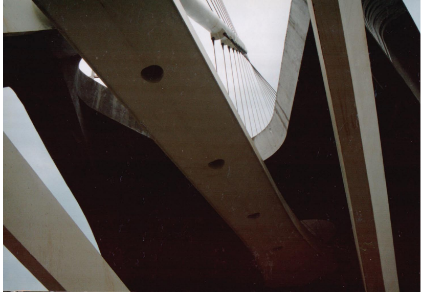
Milwaukee Art Museum under construction, 2000.
