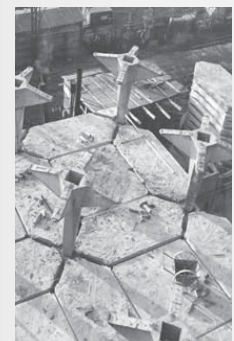
↑ The columns were prepared for upper floors. ↓ Typical partial plan.
