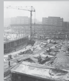
↓ Construction hoisting was done by a crane riding on a perimeter track.
