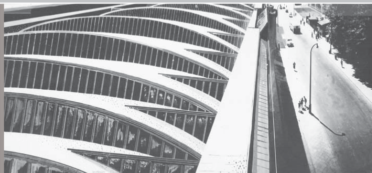
↑ The extreme depth of the trusses used to support the formwork kept member forces very low and allowed the use of small, economical sections for the members.
