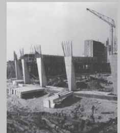
↓ These short columns are among those that balance the concrete bowl.
