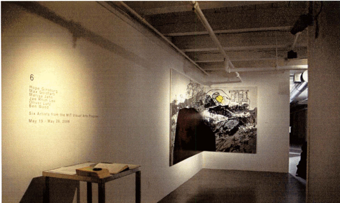
Figure 15 - Photo of gallery entrance with infrared cctv camera in upper right corner.
