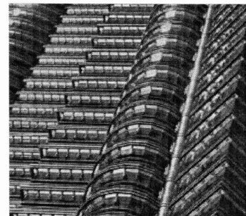
Figure 27: The Petronas Tower by Cesar Pelli Image shows the emphasis on the horizontality of the tower. - image taken from Michael J. Crosbie’s Curtain Walls
