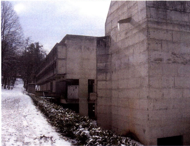
View of the cavity right before the penetration
