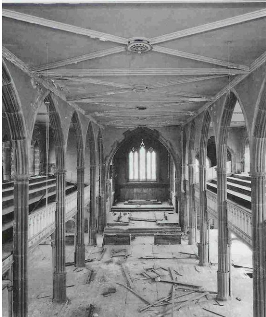
Figure 1.5: Abandoned Church, Detroit, MI
