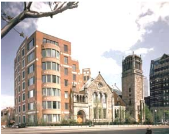
Figure 5.1: Church Court Condominiums
