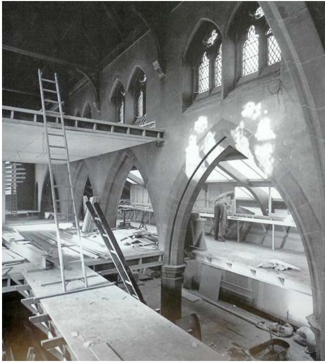
Figure 5.8: St. Michael's During Construction
