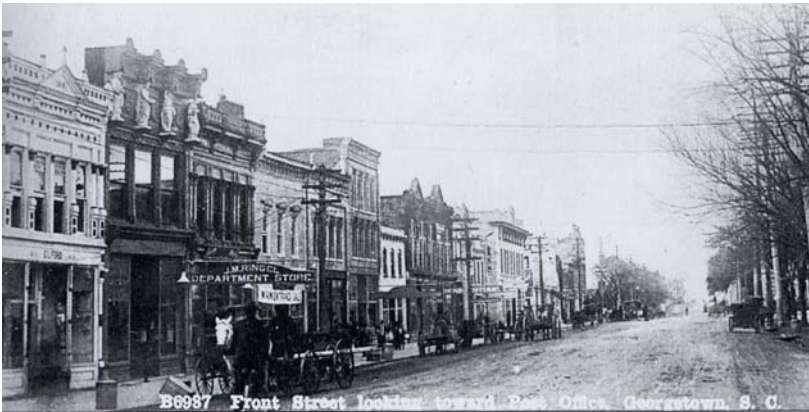
Figure 2-7: View west down Front Street.
