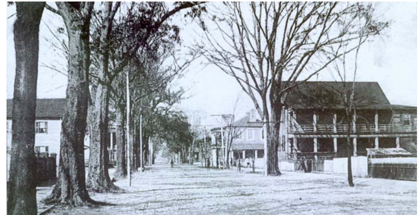
Figure 2-13: Prince Street, typical neighborhood street, 1909.
