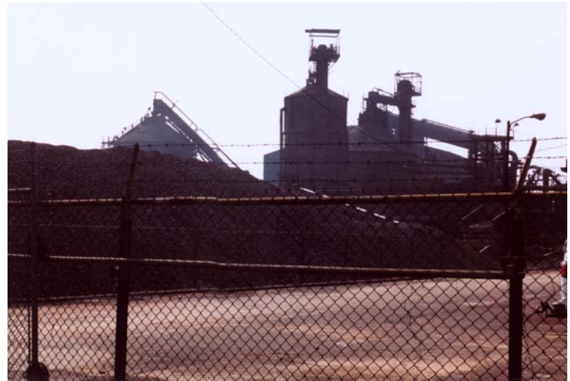
Figure 6-13: Equipment & materials in production area, north part of site.
