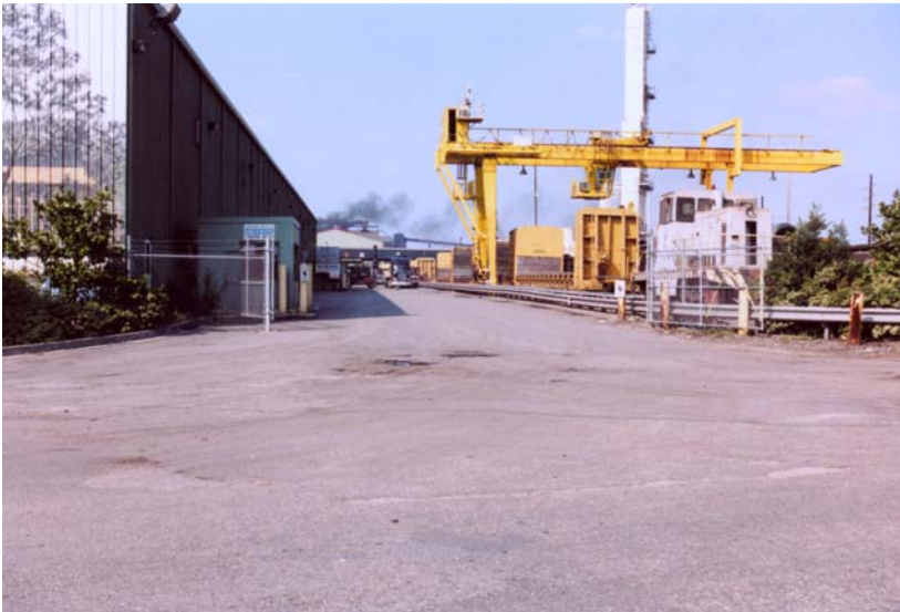
Figure 6-14: Equipment & warehouse in shipping area, south part of site.
