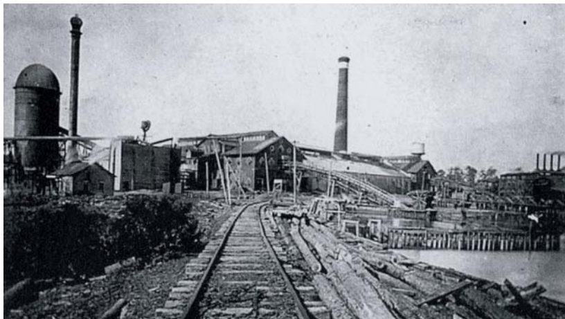
Figure 6-4: 1905 image of railroad tracks leading onto ACL site.
