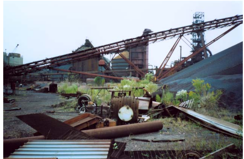
Figure 6-12: Equipment & materials in production area, north part of site.
