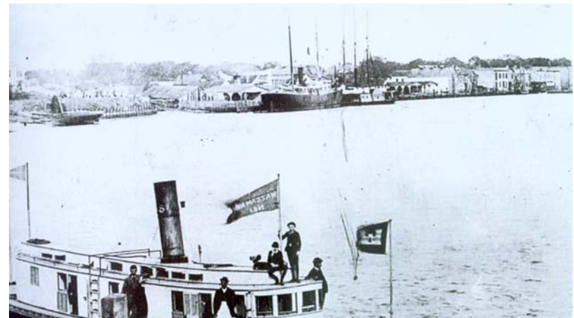
Figure 6-6: Image from ACL site towards downtown Georgetown.
