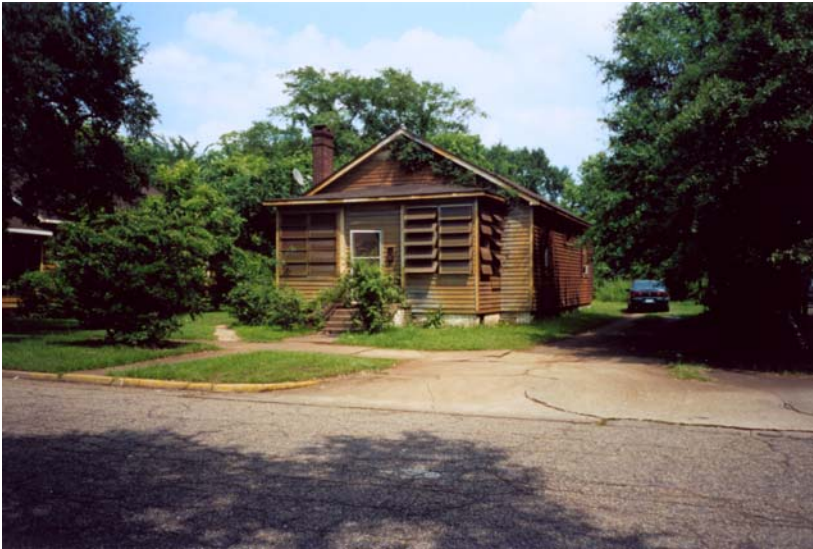
Figure 3-11: A 'rust' house in the path of the steel mill's emissions.
