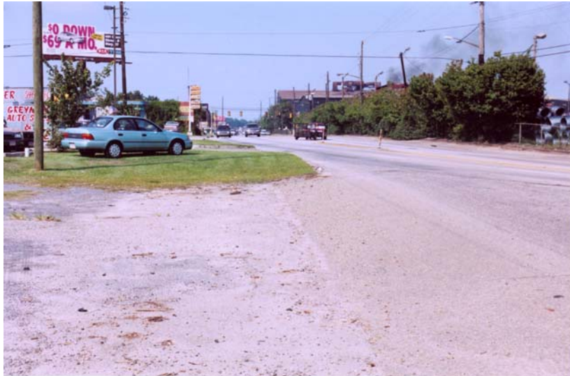
Figure 6-17: Highway 17 North, west of GSC site.
