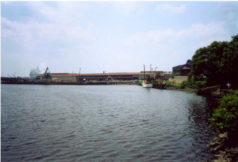
Figure 6-11: Sampit River, foreground, linear warehouse on GSC site, background.
