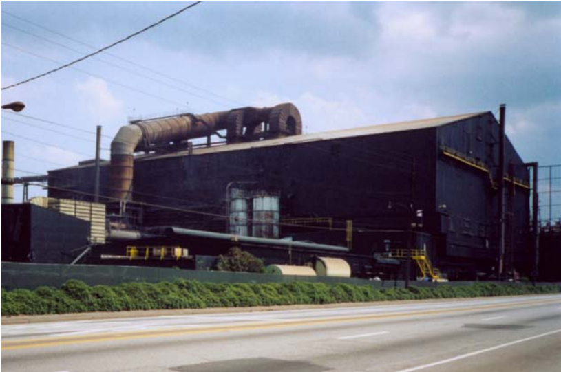
Figure 6-10: Furnace building, typical warehouse structure on GSC site .
