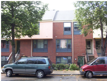
Figure 23. At the Villa Victoria development in Boston's South End, careful attention was given to providing individual entrances, as in these rowhouse flats. Duplex units are stacked over half-sunken flats.
