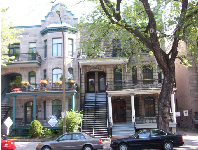
Figure 3. The street-shaping potential of superposed flats is much in evidence in this of a typical Montreal streetscape.
