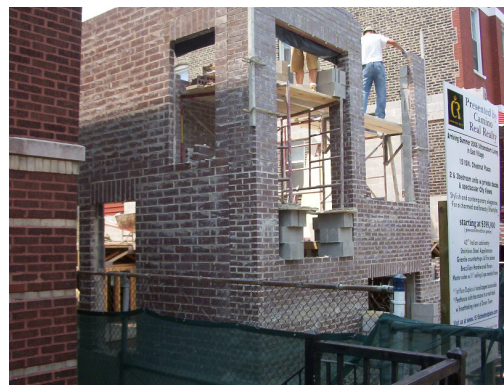
Figure 40. A typical example of modern fire-proof construction in Chicago, which is required of all residential buildings higher than two stories. The structural system is built out of concrete block, and a brick veneer is laid next to it on the exterior.
