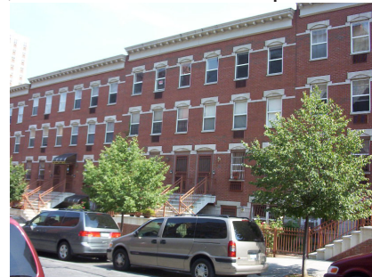
Figure 11. Newly-built rowhouse flats made to emulate the traditional brownstone scale and appearance of the surrounding neighborhood, Harlem, Manhattan.
