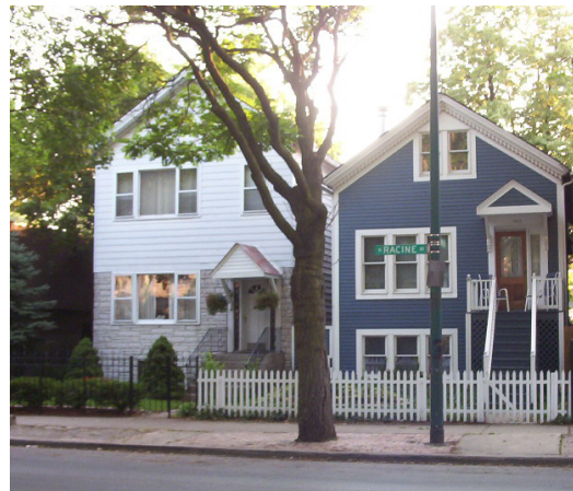
Figure 32. Typical 1910s-era workingman’s cottages, Ukrainian Village, Chicago. Such housing stock is commonly targeted by developers for acquisition, teardown, and replacement with new construction three-flats.
