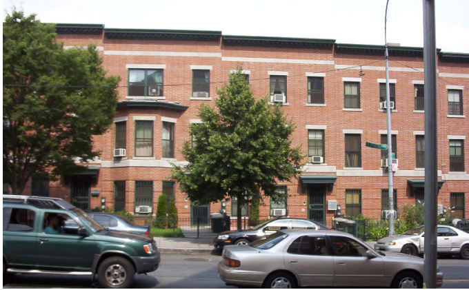
Figure 36. An example of three-family houses built under New York City's Housing Partnership New Homes program by the Hudson Companies. These rowhouse flats are adjacent to the Atlantic Center mall just outside of Brooklyn's Central Business District.
