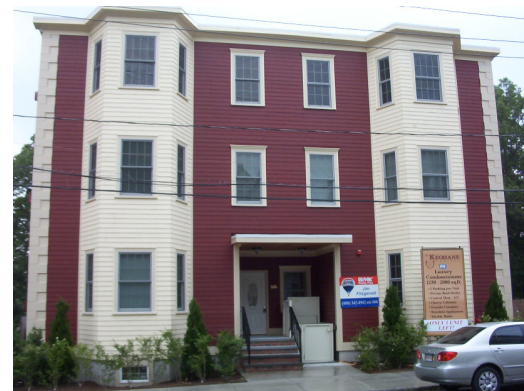
Figure 41. A recently-built six-family house in the Neponset section of Dorchester, Massachusetts uses a wheelchair lift (bottom center, to the right of the staircase) to provide wheelchair accessibility to the two ground-floor apartments.
