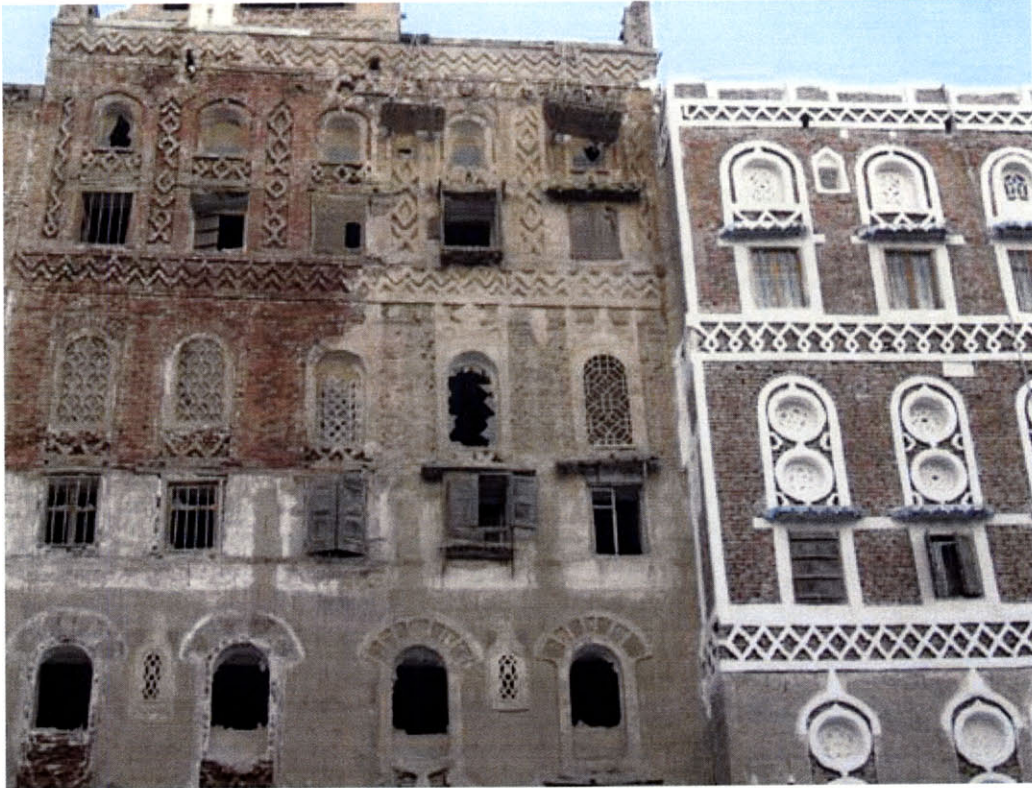
Figure 40 Houses at al-Abhar Square during the Ministry of Culture's white-washing project. The façade on the left has been scraped; plaster on the right has been applied against a straight-edge.
