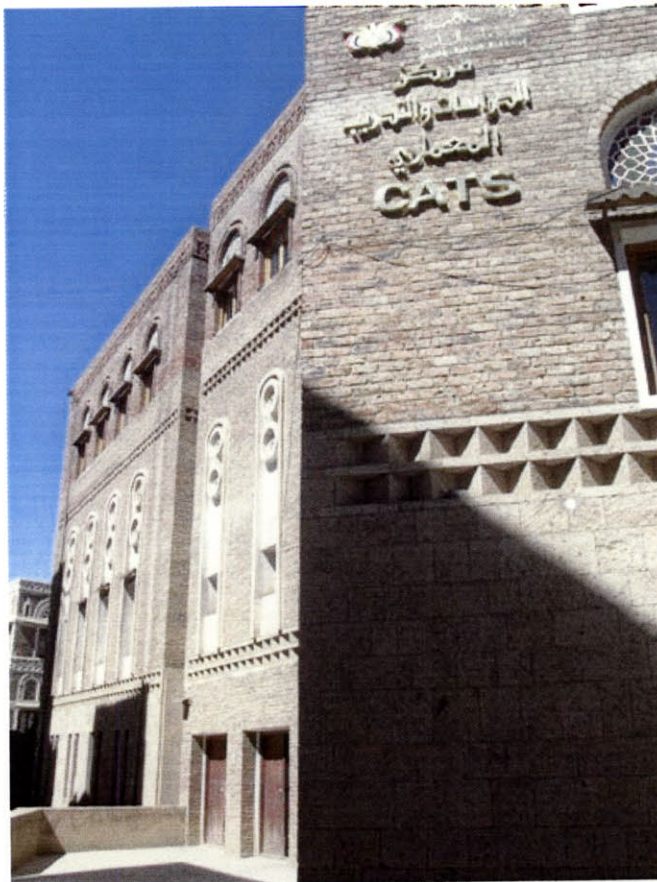
Figure 35 The Center for Architectural and Technical Studies (CATS), designed by Quaroni Bonifica.
