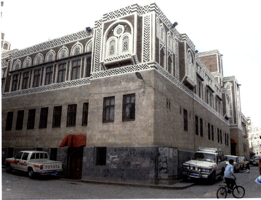
Figure 14 Suq al-Baqar clinic, southeast corner.
