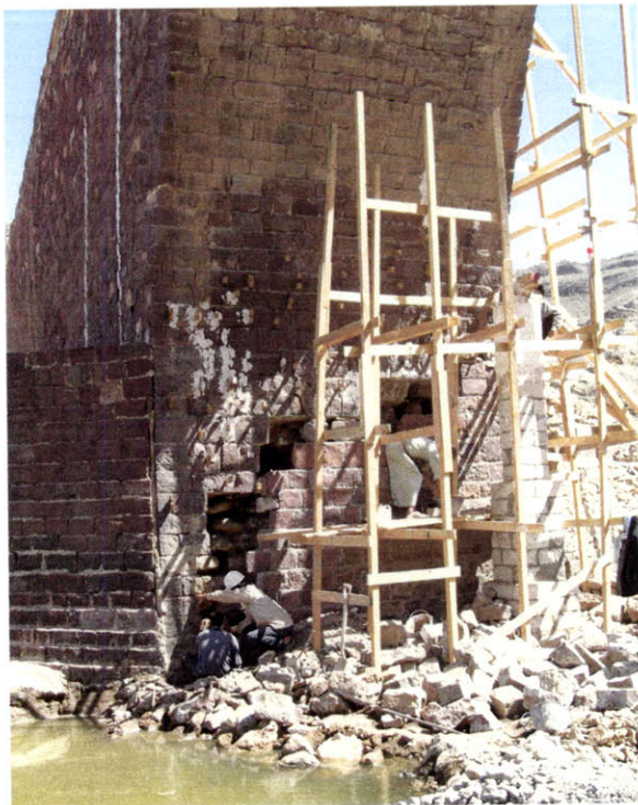
Figure 27 The Rasulid bridge at Damt, to the southeast of Sana'a. In late 2004 the bridge was being restored by usta 'Abdullah al-Rawdhi, under the supervision of the Social Fund for Development. The wooden device in the middle of the image was constructed by al-Rawdhi to calculate the arch of the bridge.
