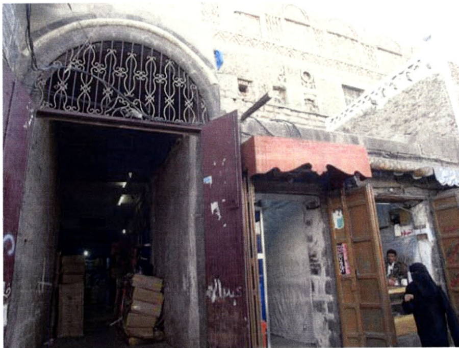
Figure 22 Samsarat al-Baw'ani, south entrance after renovation.
