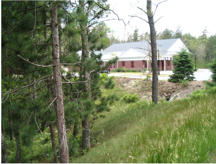
Plymouth fire station and naturally vegetated depression, which took the place of a conventional detention basin.
