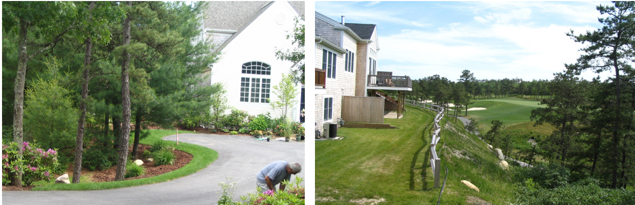
(from left) Rain garden positioned to capture runoff from driveway; Homes placed along ridge of hill to take advantages of golf course and forest views and aid with drainage.
