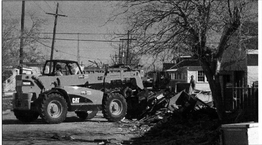
Image 28: Contractors clearing debris off the streets
