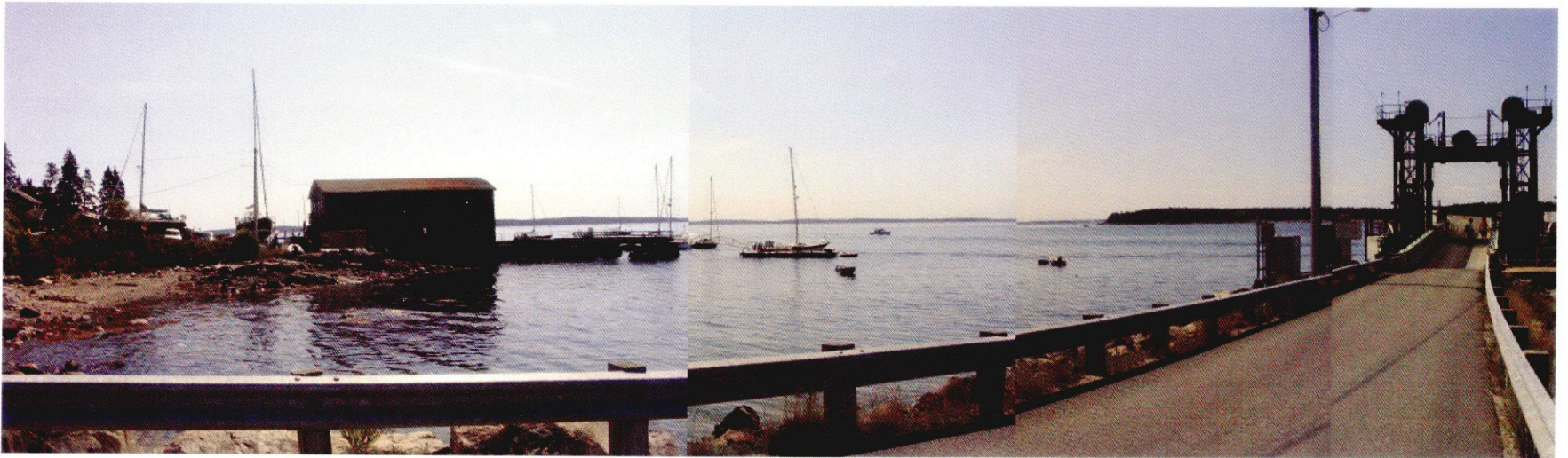
The Swan's Island ferry landing, secondary public access point
