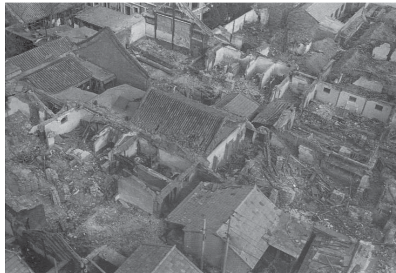
Fig.0.9 Rapid demolition of hutong neighborhood
