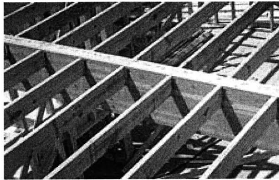
Figure 19: Floor Glulam Beams
