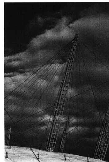
Figure 10: Masts of the Millennium Dome (Koch et al., 2004)
