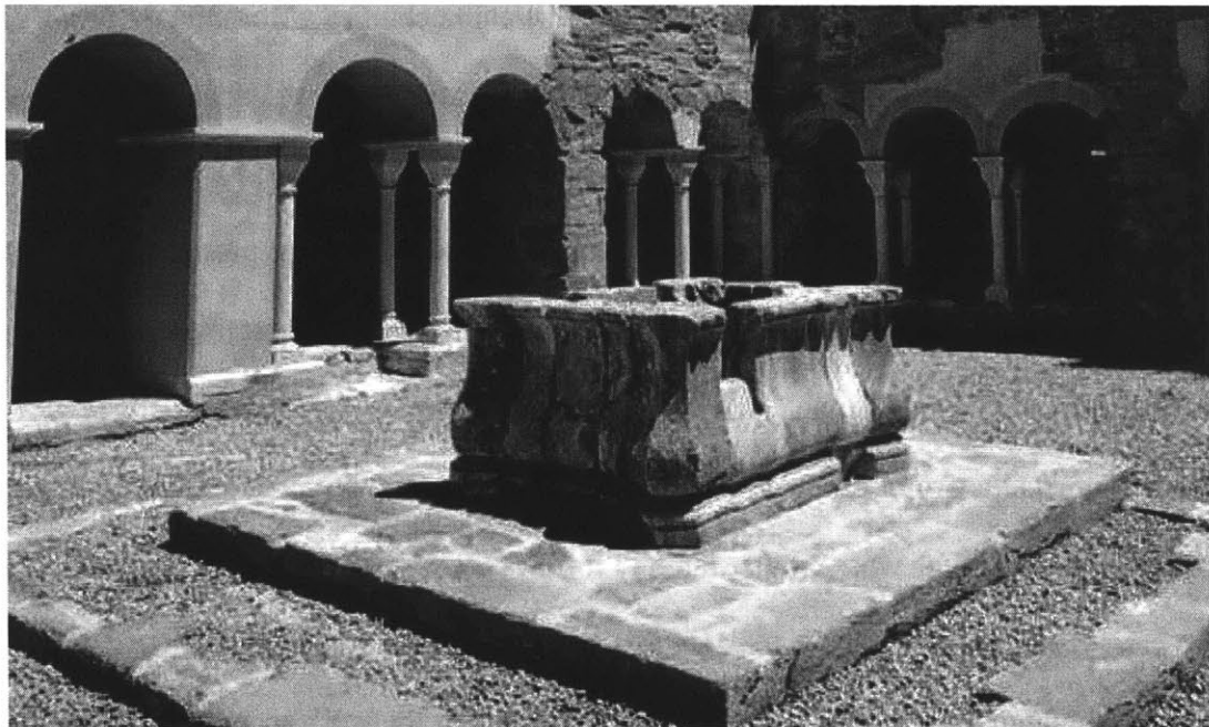
Fig. 1. Cloister of the Monastery of Sant Pere de Rodes. This is an example of a purist restoration: the added parts are visibly differentiated from the original ones.
