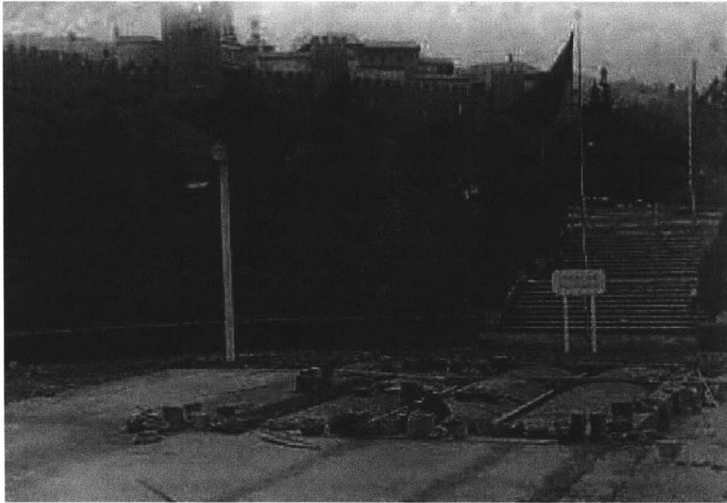
Fig. 17. Construction of the Pavilion's foundations by means of Catalan vaults, 1929.
