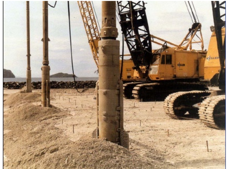
Picture 17 Vibrocompaction machines
