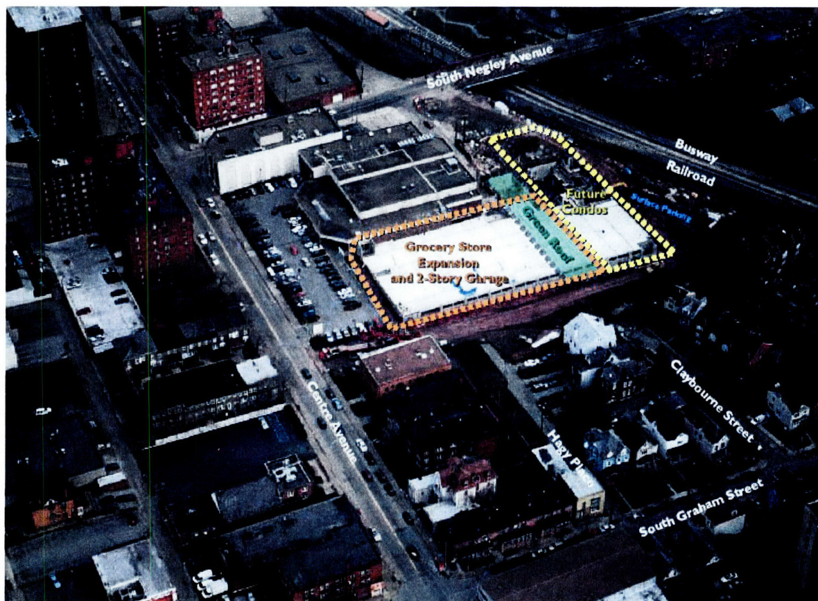
Figure 6.8 Negley Station Grocery Store and Condominium Development
