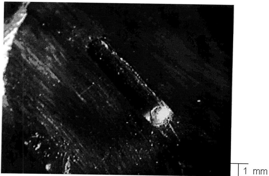
Single cracking appearance at the second cycle (A2)
