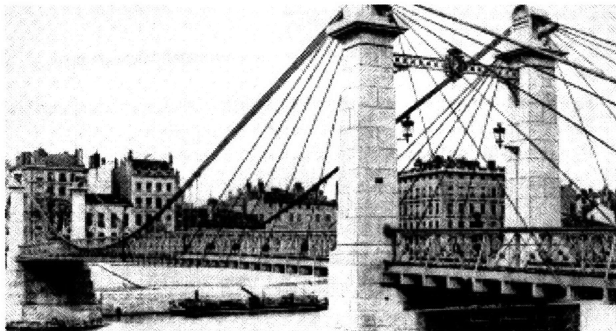
FIGURE 2.10: SAONE RIVER BRIDGE
