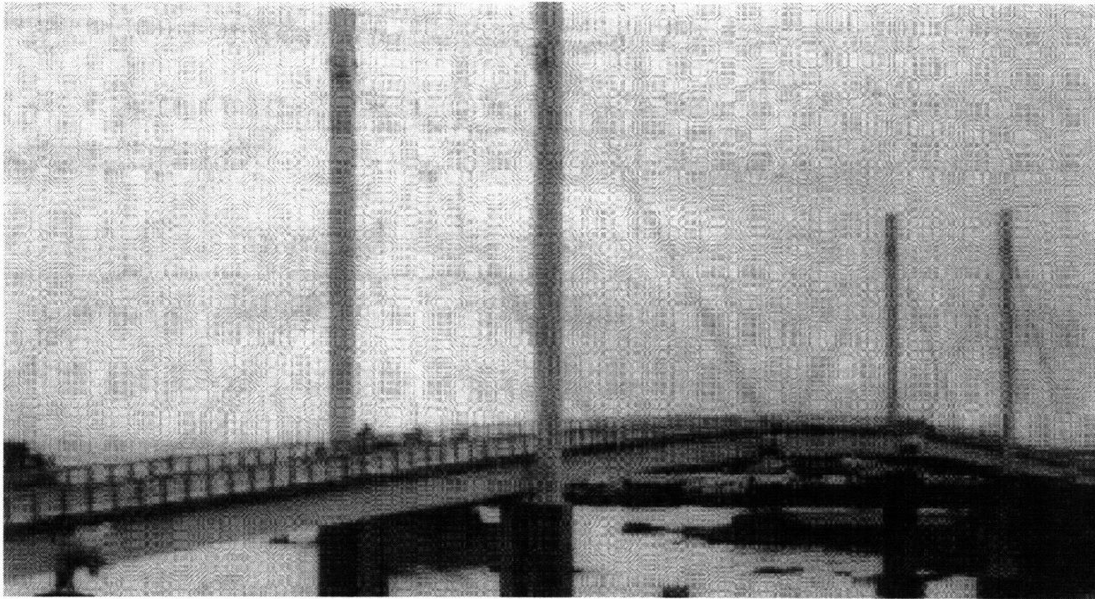
FIGURE 2.30: SITKA HARBOR BRIDGE
