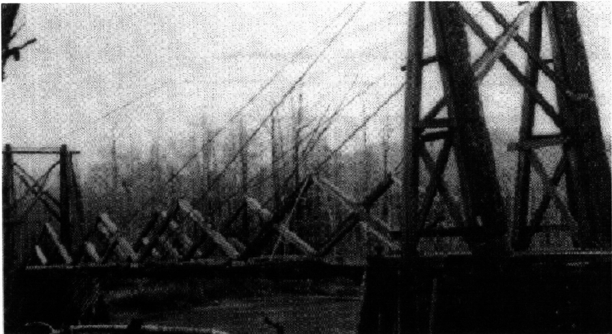
FIGURE 2.28: QUINALT RIVER BRIDGE
