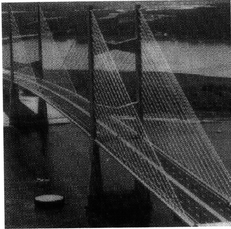
FIGURE 2.32: DAME POINT BRIDGE
