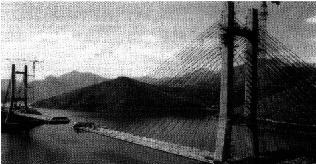
FIGURE 3.12: BARRIOS DE LUNA BRIDGE
