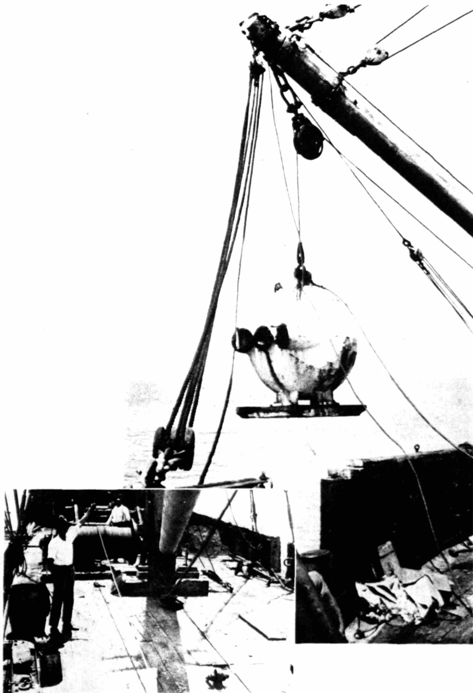
Upper: The bathysphere poised over the water with Beebe and Barton inside, ready for one of the deep sea dives. Lower: The Arcturus winch and the heavy cable, with John Tee-Van in charge of the deck crew.
