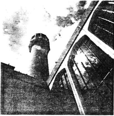
Fig. 4.18 View of the minaret and the precast concrete panels.
