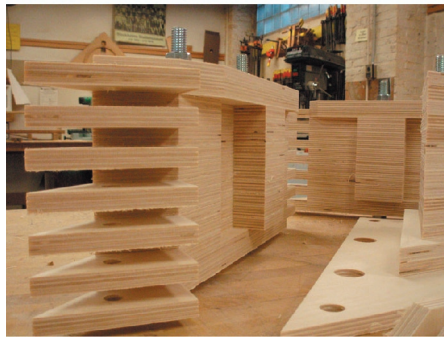
Final Formwork Prior to Casting
