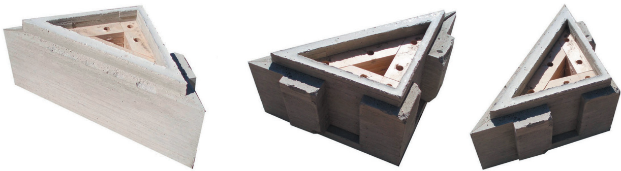
Concrete Formwork with Exterior Formwork Removed
