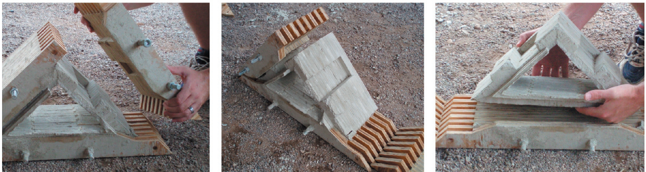
Removing Exterior Modules
