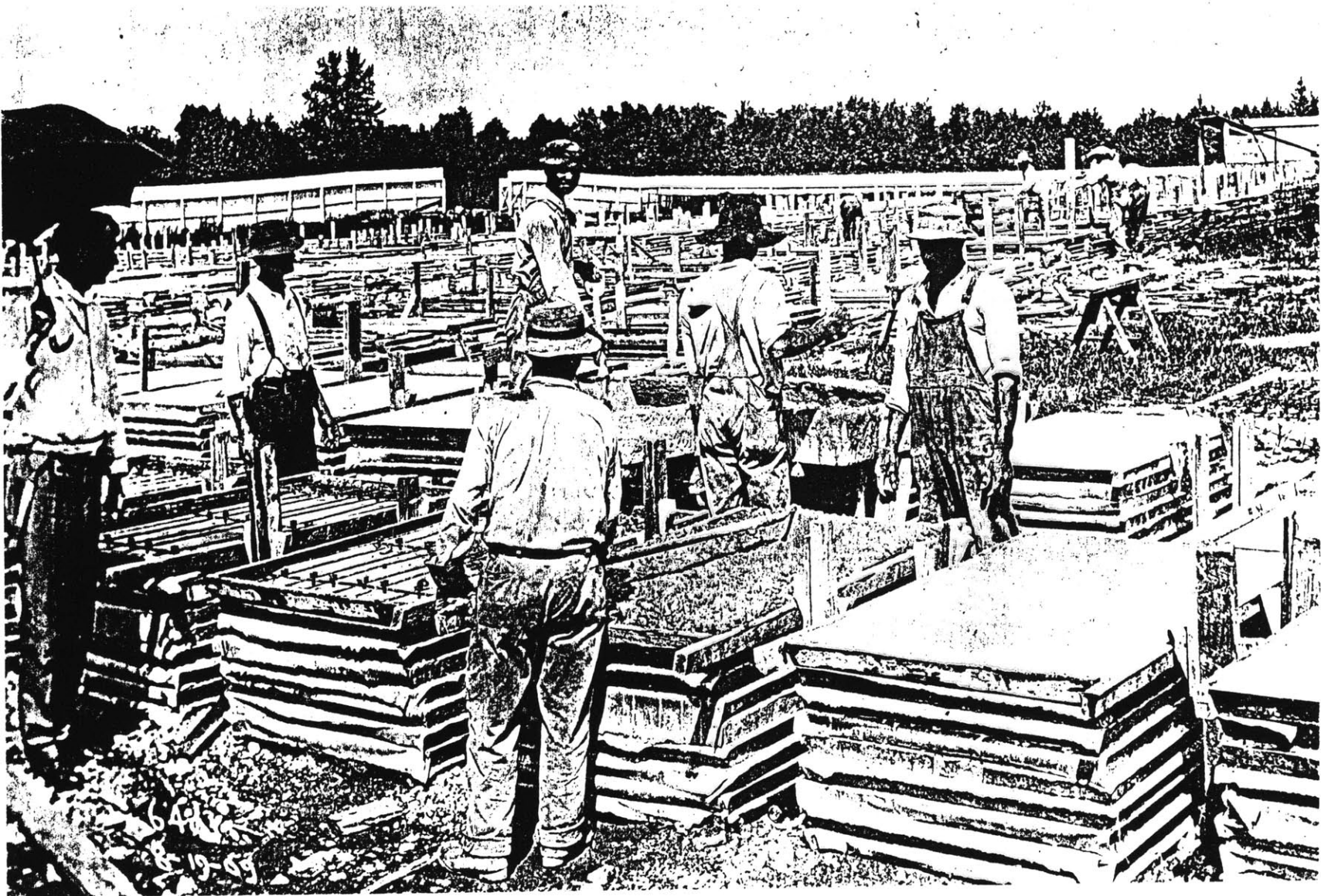
Slab concrete production, construction site of Harbison-Walker Refractory, 1909. Built by Robert Cummings. Cummings Collection Photo Albums, Mechanical and Civil Engineering, Smithsonian Institution.
