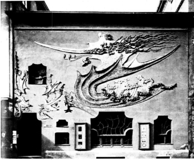
Fig.4.8: August Endell, Exterior view of Elvira Photography Studio, Munich, 1898.
