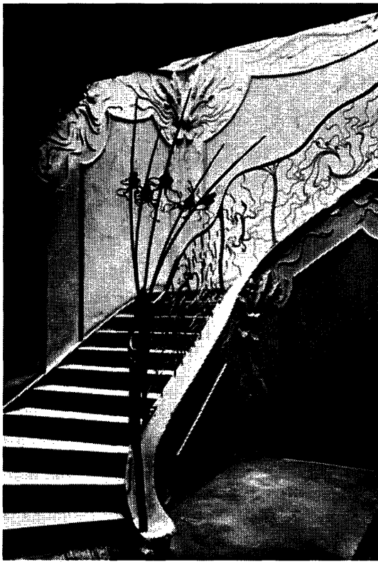
Fig. 4.15: August Endell, Interior view of stairs, Elvira Photography Studio, Munich, 1898.
