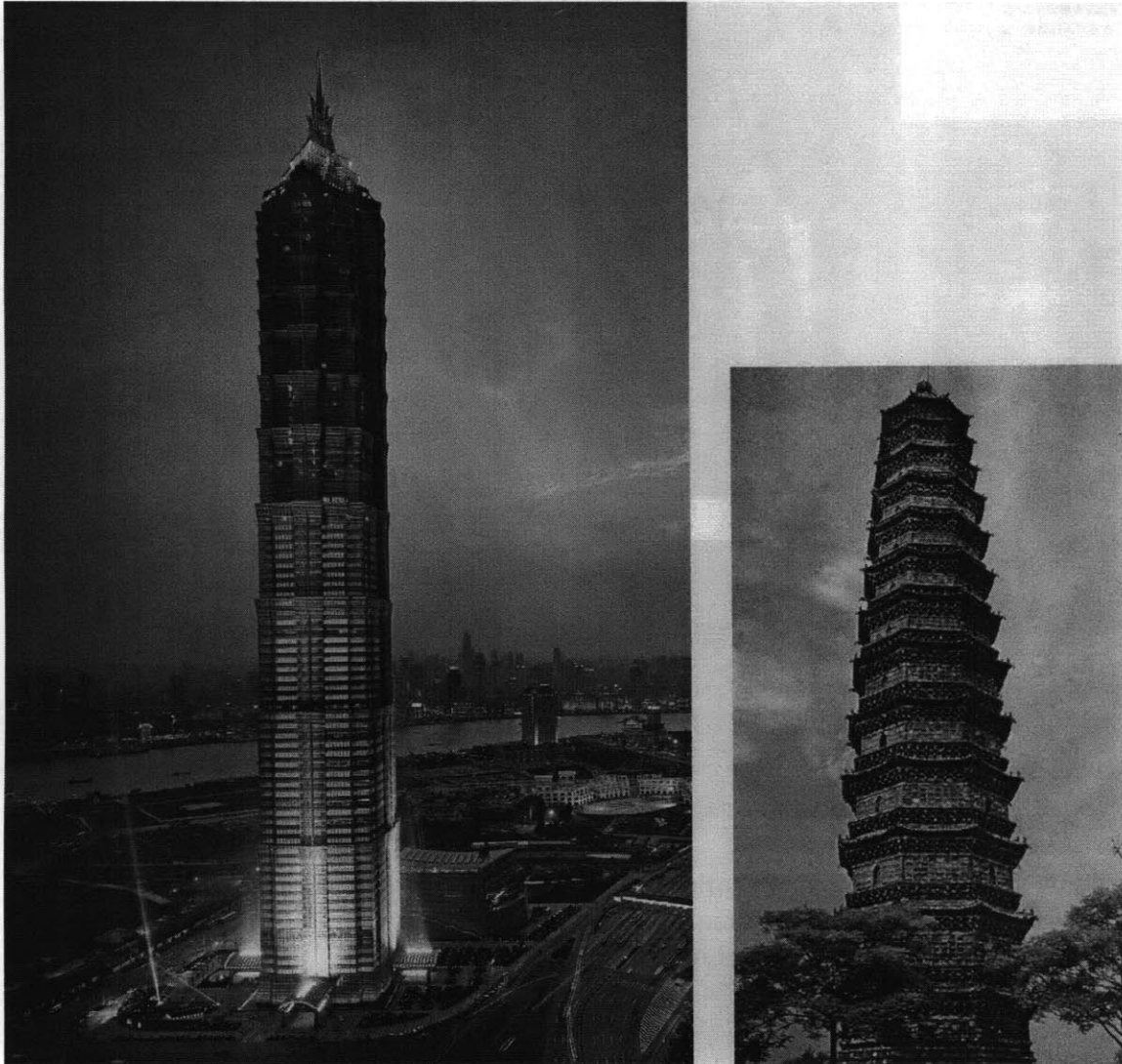
Figure 18: Left Kaifang Pagoda, and Right Jin Mao Building. Photograph: Wang Xuyuan
