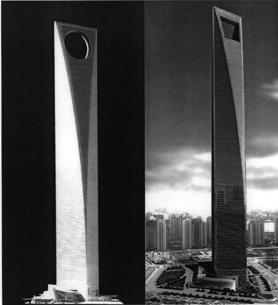
Figure 19: Left Model of the World Financial Center as original designed. Right A Rendering of the building after the circular opening on the top was replaced by the rectangle. Photographs: Kohn Pedersen Fox International
