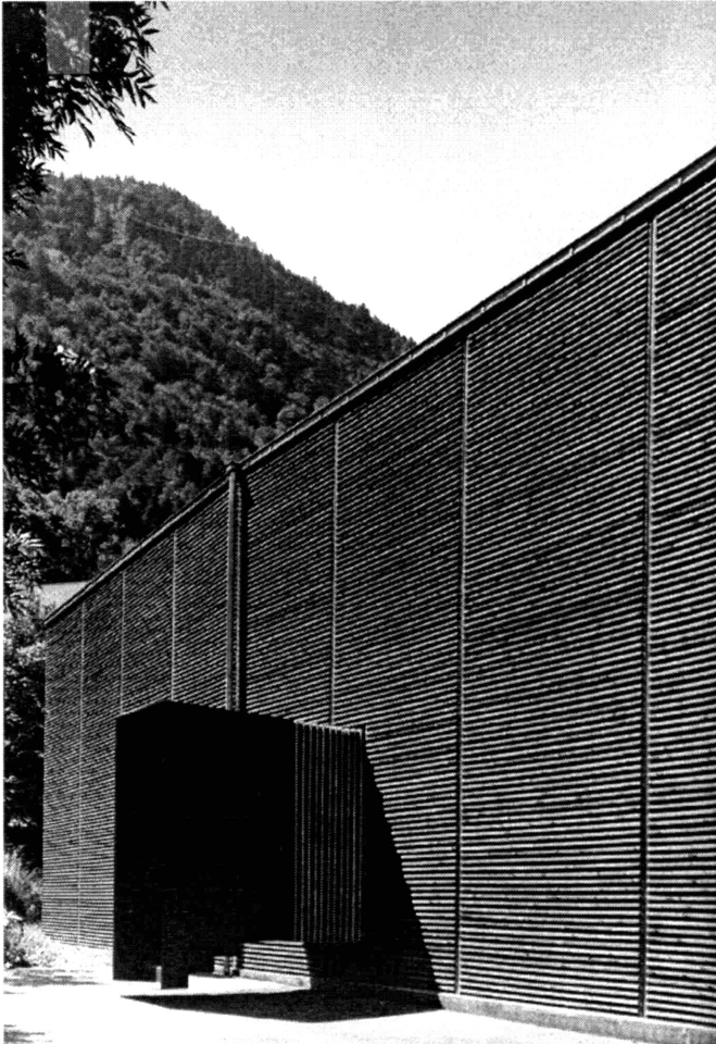
Fig 2: Peter Zumthor, Shelters for Archeological Site. Near view.
