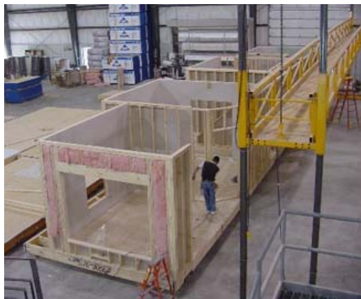
Figure 9: Prefabrication at Warehouse
