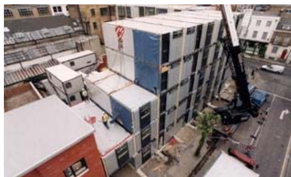
Figure 10: Stacked Modular Units
