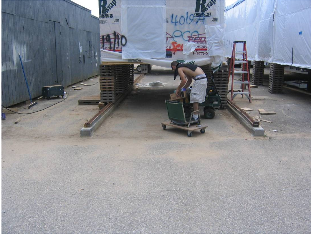
Epoch Homes Factory Pembroke, NH
