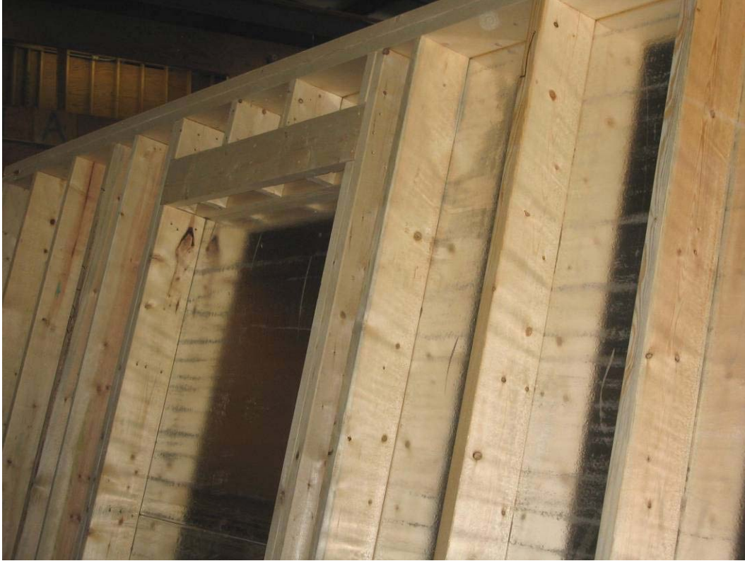
Epoch Homes Factory Pembroke, NH
