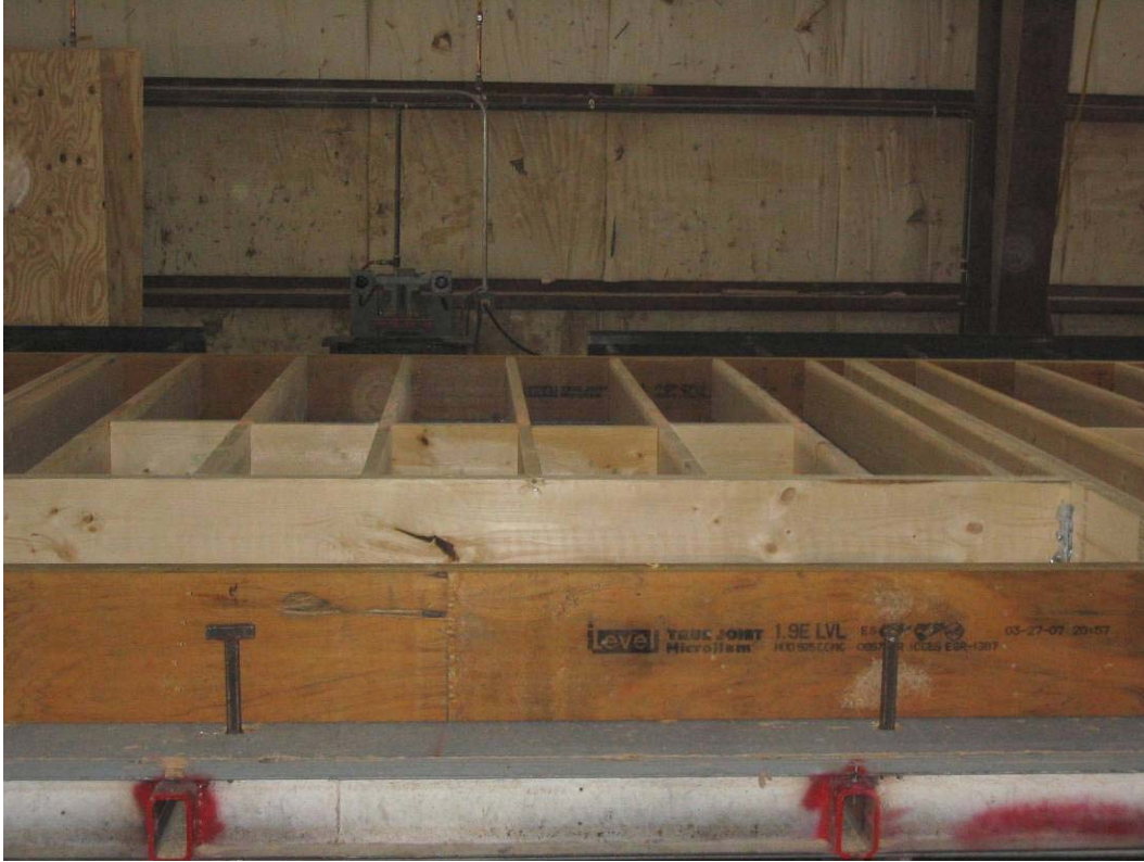
Epoch Homes Factory Pembroke, NH
