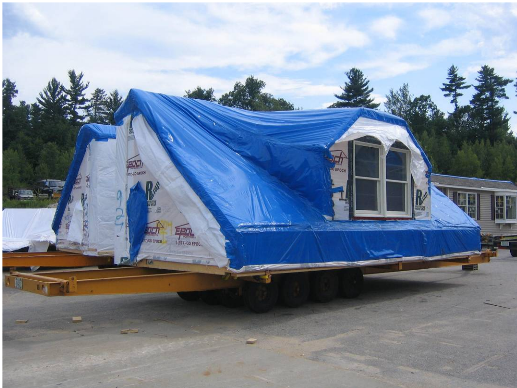
Epoch Homes Factory Pembroke, NH
