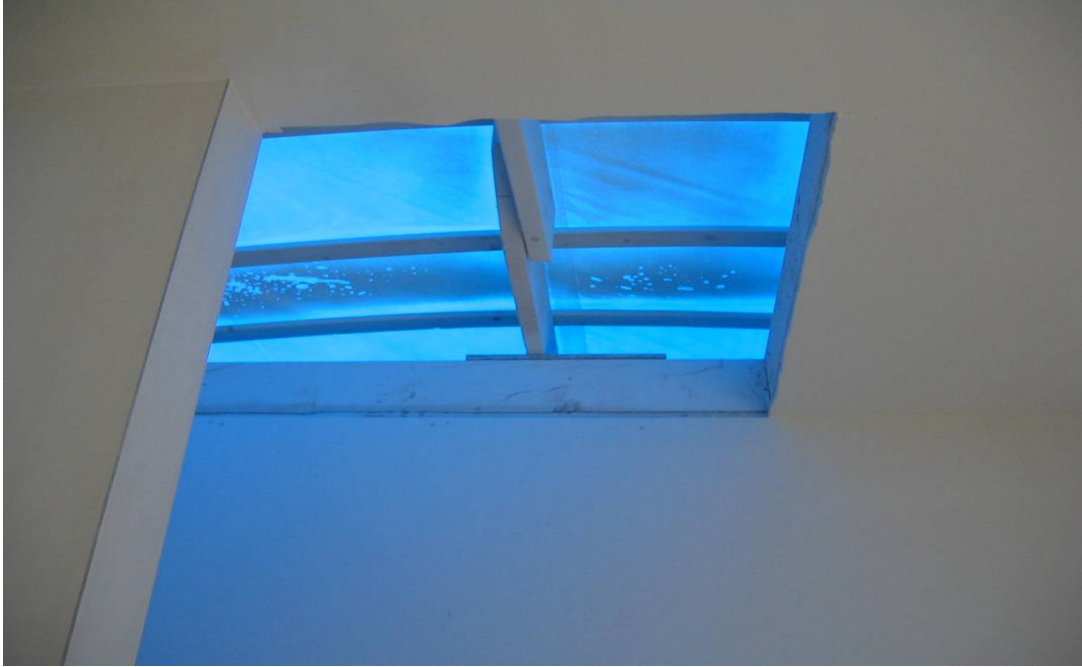
Epoch Homes Factory Pembroke, NH
