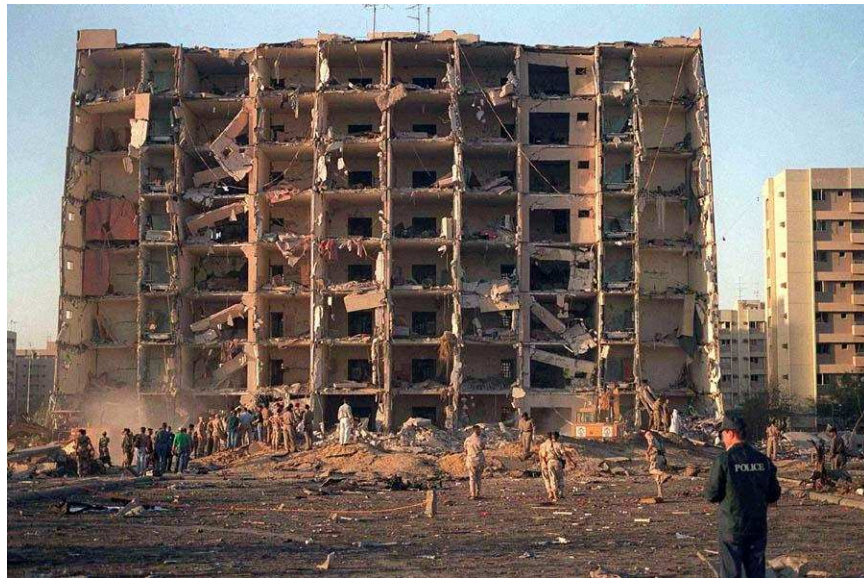
Figure 1-2: The Khobar Tower in Saudi Arabia after the terrorist attack of June 25, 1996 [74].
