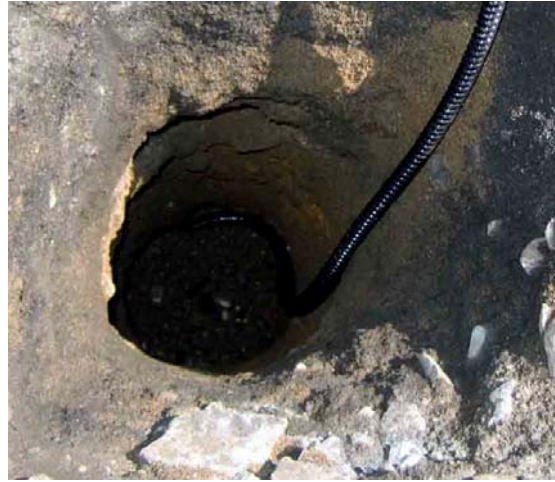
Figure 6-7: Backfilling the piezometer with Insitu soil filling.
