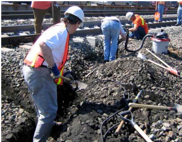
Figure 6-5: Trench digging
