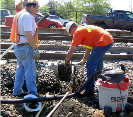
Figure 6-6: Augering until 1.8m depth for deep piezometer installation.
