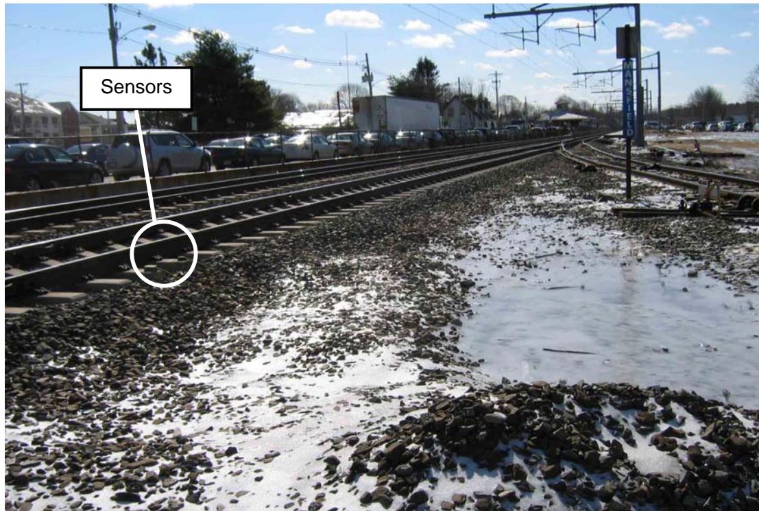
Figure 8-5: Frozen ground, picture dated 16 Feb 07 (day 239).
