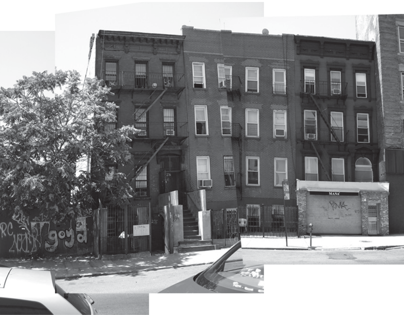
The rear of the building on South 5th Street viewed from across the street.
