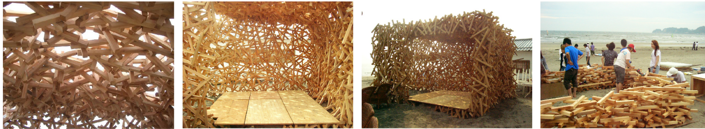
A9/ LAYERING_ One unit repeated on several offset layers (000studio, Algorithmic Space)
