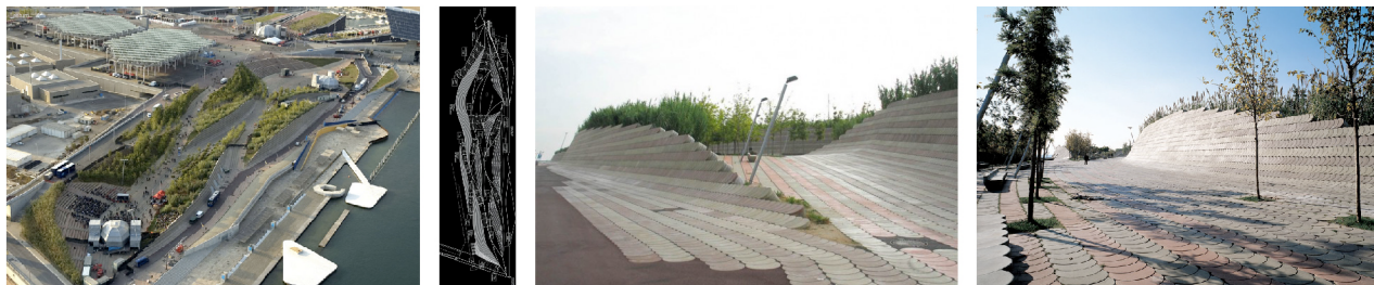
B4/ TOLERANCE_ Single module repeats non-uniformly with deformations taken up by tolerance between tiles (FOA, Coastal Park)
