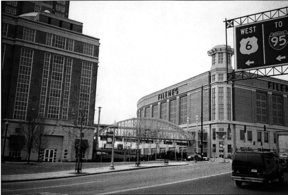
Exhibit 5: Post Revitalization Skybridge link between Providence Place Mall and Westin Hotel
