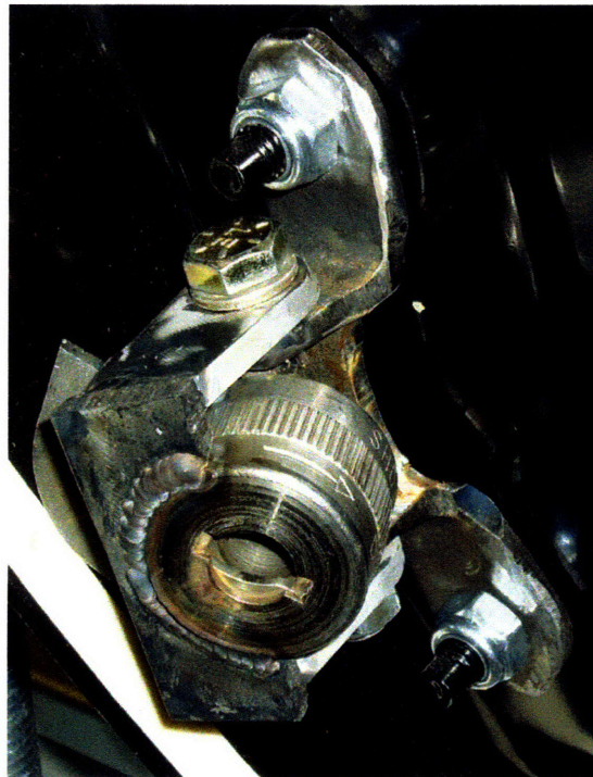
Figure 3-8: Socket welded to hinge and bolted to door frame
