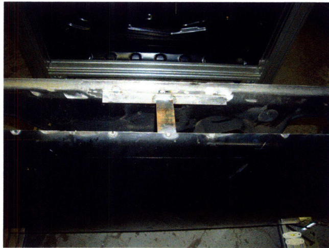
Figure 3-2: Reinforcement piece welded between two door panels
