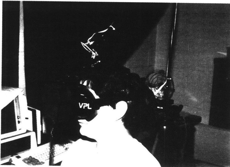
**Figure 2.4 - Subject Wearing Head-Mounted Display, with Head-Tracking Linkage**
