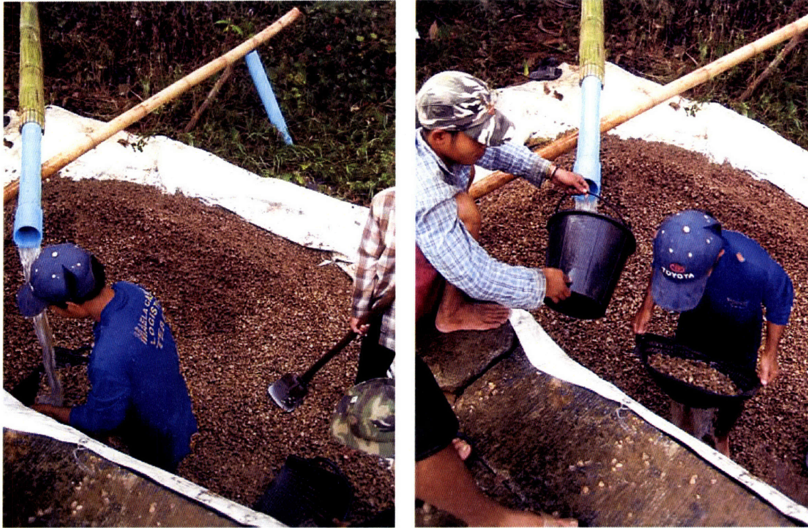
Figure 6-1: Cleaning the HFRF media. (L) Shows the gravel removed from the filter, (R) show the workers cleaning a basketful of gravel with the diverted water supply.
