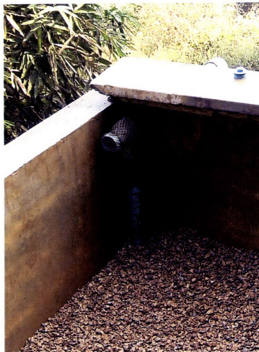
Figure 7-1: Slotted outlet pipe..
