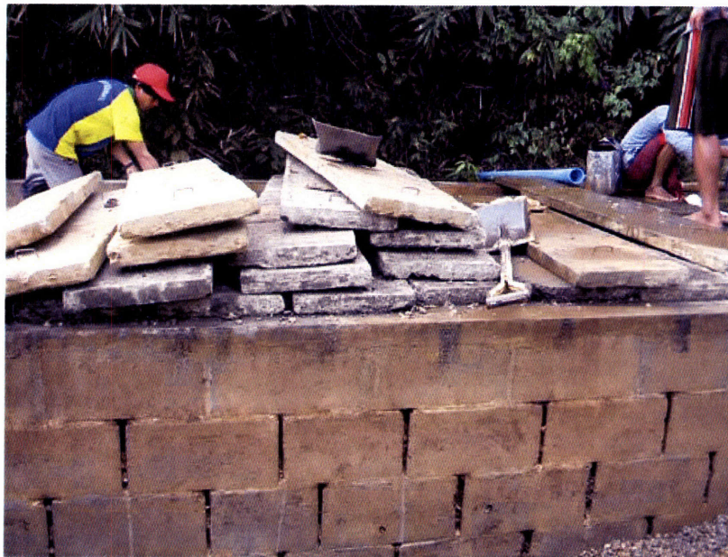
Figure 3-7: Internal wall of SP-10 HFRF.
