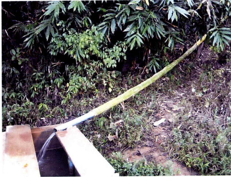
Figure 3-8: Inflow pipe to SP-10 HFRF.
