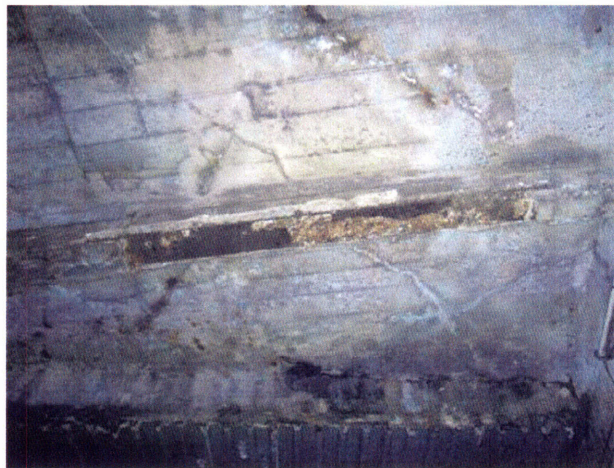
Figure 4-9, Ashmont Station, Red-line, Boston, MBTA (Russell 2007)
