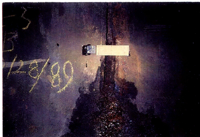
Figure 4-13, Crack Monitoring Gage, Chicago (Russell 1989)
