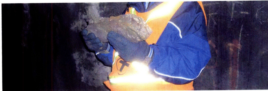
Figure 4-18, Concrete Spall Fell on the Track at Ashmont Station, Red-line, Boston MBTA, (Russell 2007)
