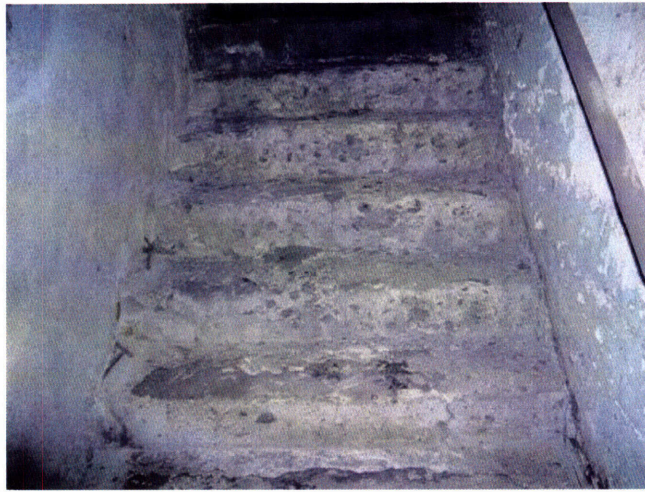
Figure 4-20, Emergency Exit Stairwell, Andrew Square, Red-line, Boston, MBTA, (Russell 2006)
