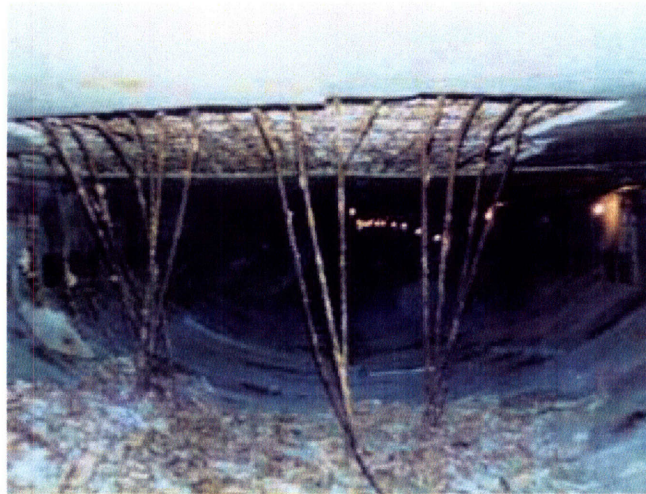
Figure 4-22, Sumner Tunnel, Boston, (Russell 1989)
