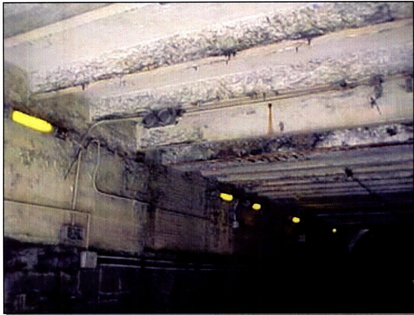
Figure 4-3, Roof of Park Avenue Tunnel, New York City, (Russell)
