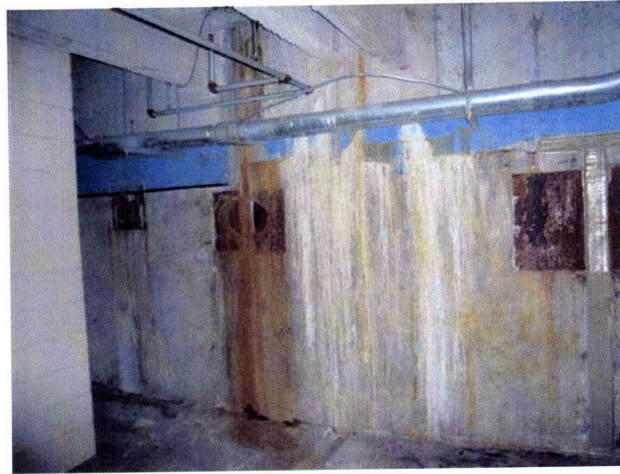
Figure 4-17, Waterfront Underground Parking Garage, Boston, MA, (Russell 2007)
