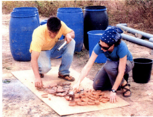
Figure 51 Carl Allen (Peace Corps) and the author breaking ceramic pottery pieces for the pilot HRF
