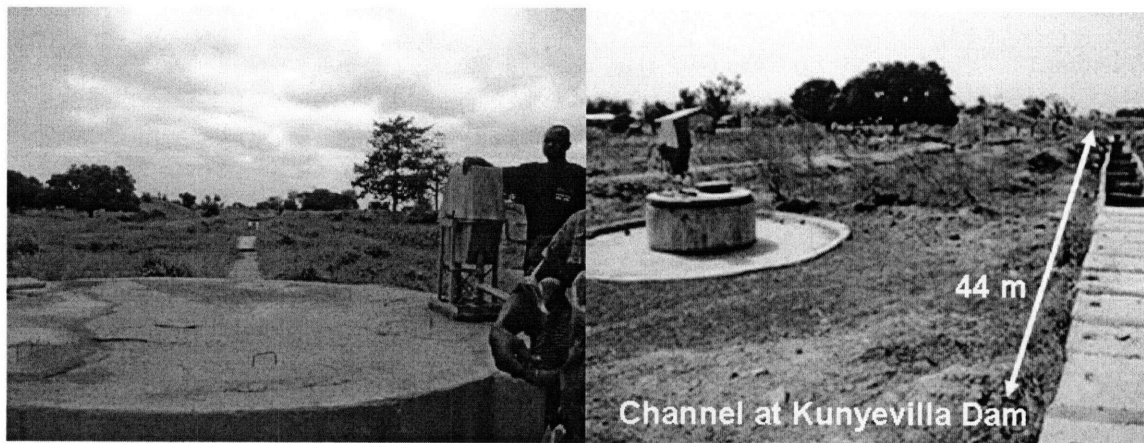
Figure 76 Kunyevilla Dam cistern and channel in the rainy season (left) and the dry season (right) Photo Credit: Kelly Doyle (2007) (left)
