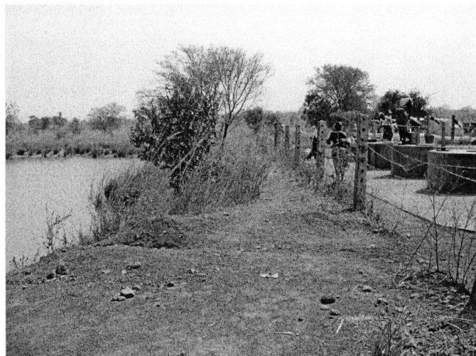
Figure 36 Gbrumani Dam and hand pumps, Tolon District
