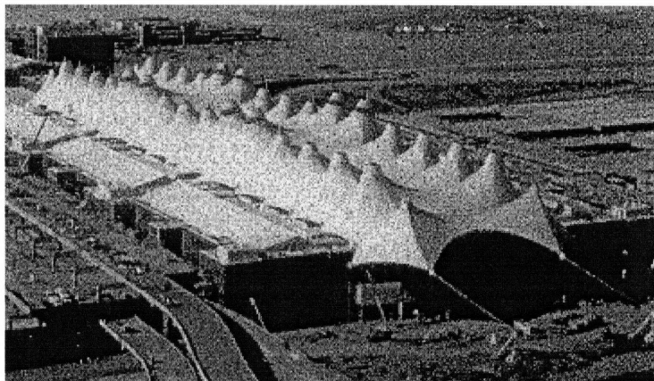
Figure 3-1: Denver International Airport (Berger, 1999)
