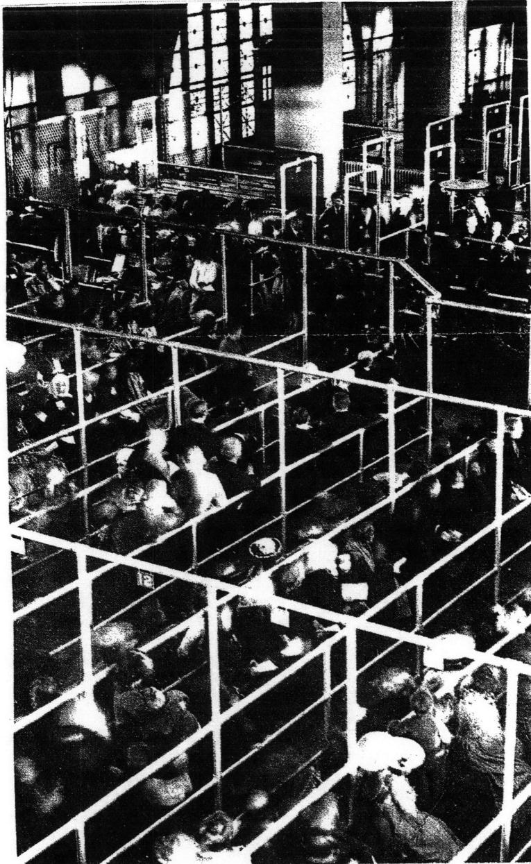
Fig. 5. Pipe rail enclosure at Ellis Island
