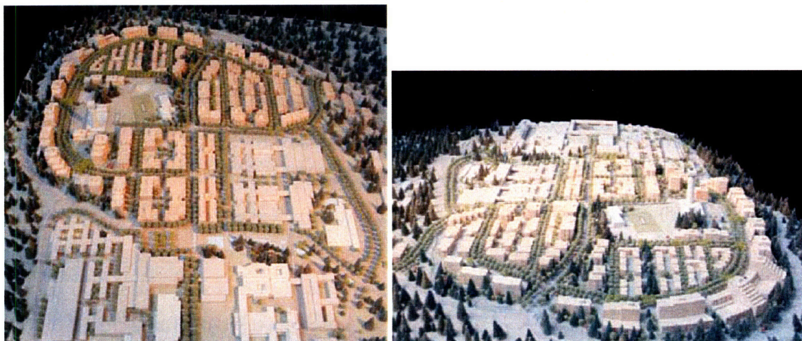
Figures 3.38-3.39: These images of a model of the UniverCity project clearly show the way the development responds to the topography of the mountaintop. While Erickson’s campus plan was terraced into the mountaintop and emphasized horizontality, the UniverCity plan takes more liberties with towers and adds an element of verticality to the site. The development is also designed to fit closely within the confines of the ring road. (Source: Urban Design & Master Plan for UniverCity: The Community at Simon Fraser, p. 23)
