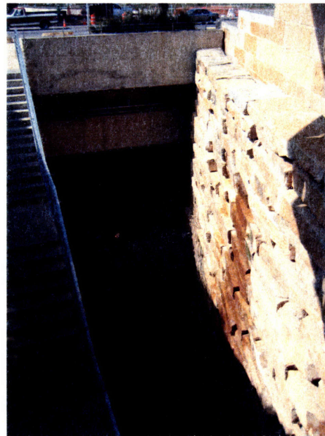
Air conditioning condensate falls from rocks composed to look like a naturally occurring formation in Austin's hill country Photo: Kristen Hall
