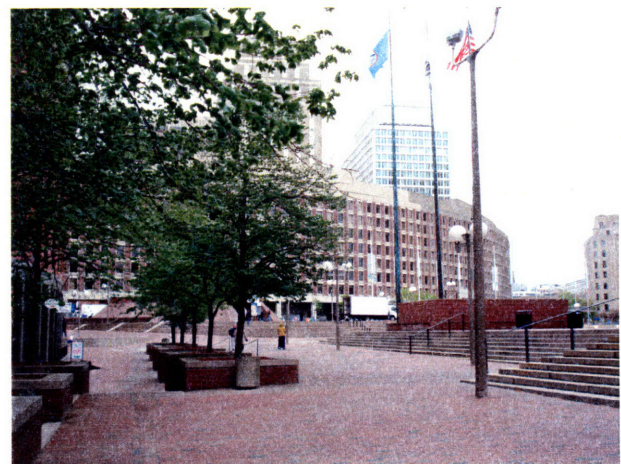
The plaza is an unending obstacle course for those who may have trouble with climbing stairs. Photo: Kristen Hall
