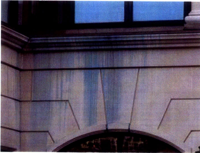
A closeup shot of the new theater weathering
