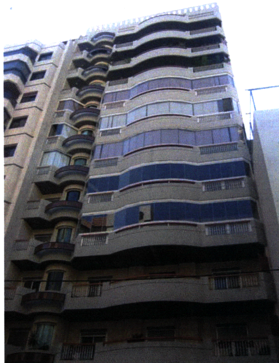
Figure 4.9: One of the new, modern, large, and relatively more expensive buildings in Ras el Nabaa.
