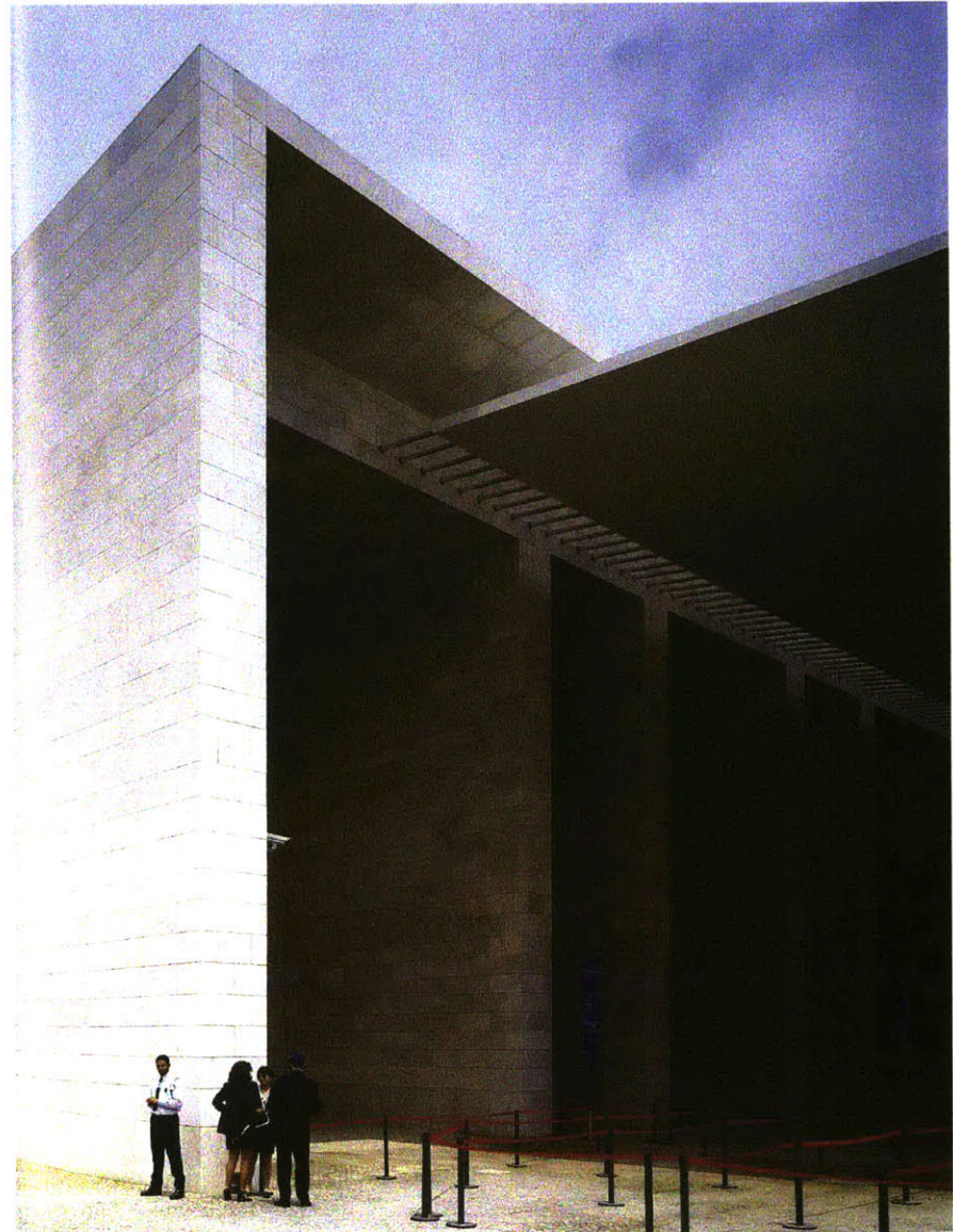
Portuguese Pavilion details showing reinforced concrete shell roof
