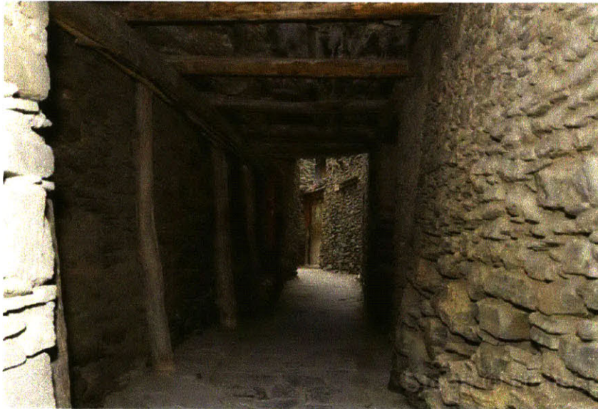
covered walkway, showing partially embedded wood columns and beams
