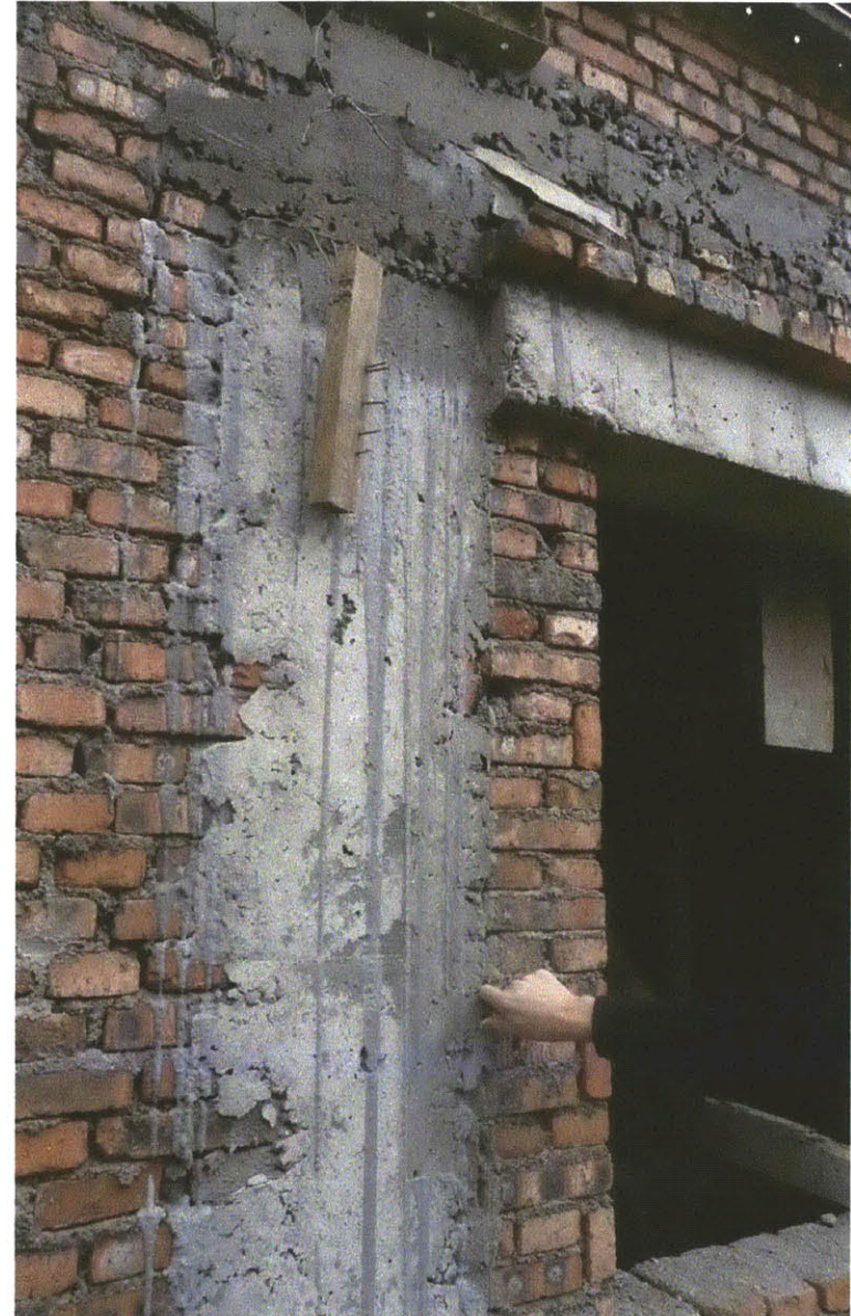
cast-in place column and precast-lintel
