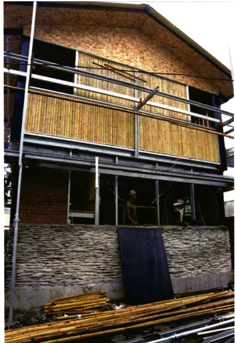
lightweight steel framed home with infill of stone, brick, bamboo and plywood
