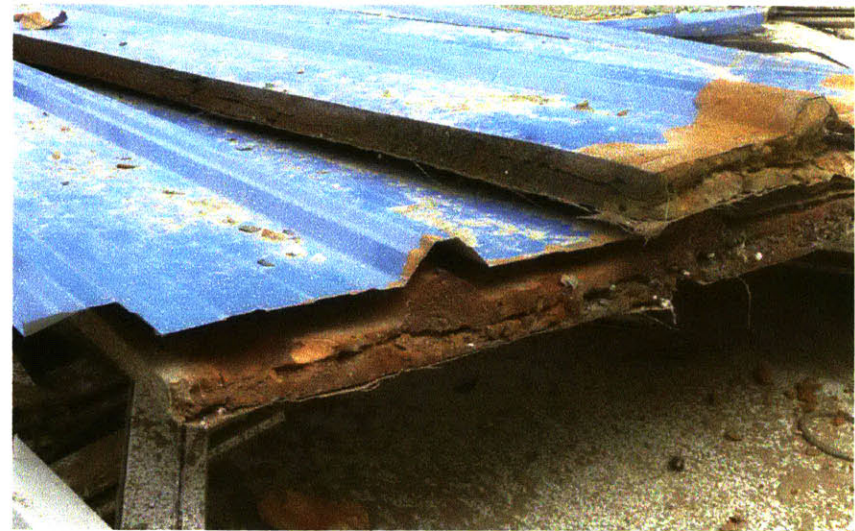
typical lightweight roofing material
