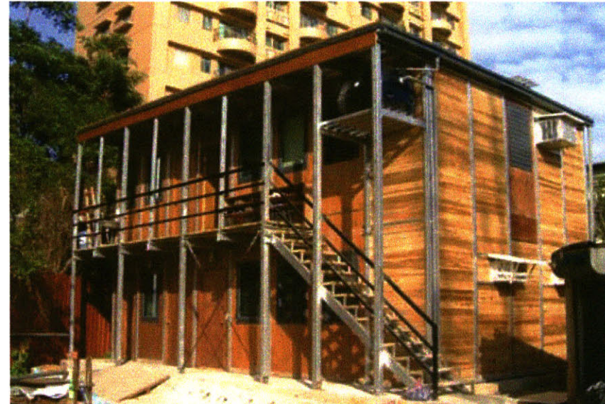
house by Hsieh Ying-Chun using lightweight steel exterior walkway system
