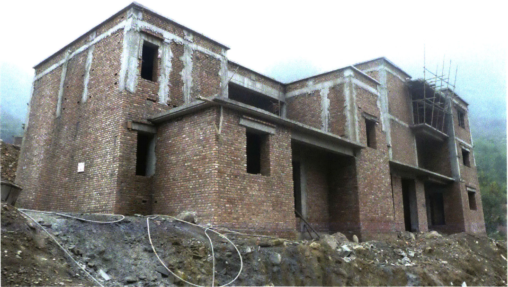
Beichuan county housing project under construction
