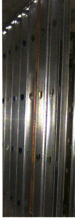
light steel framing
