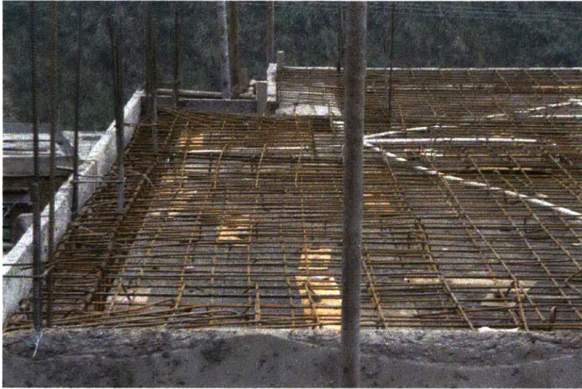
cast in place floor slab
