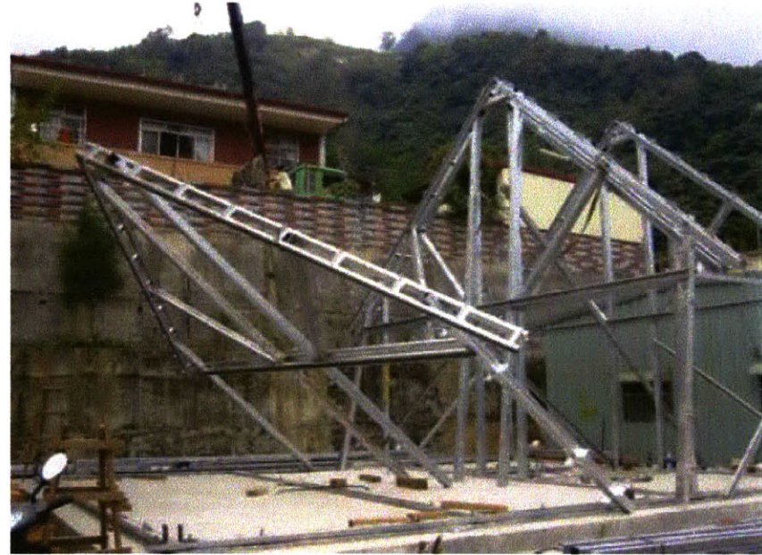
lightweight steel bents being erected
