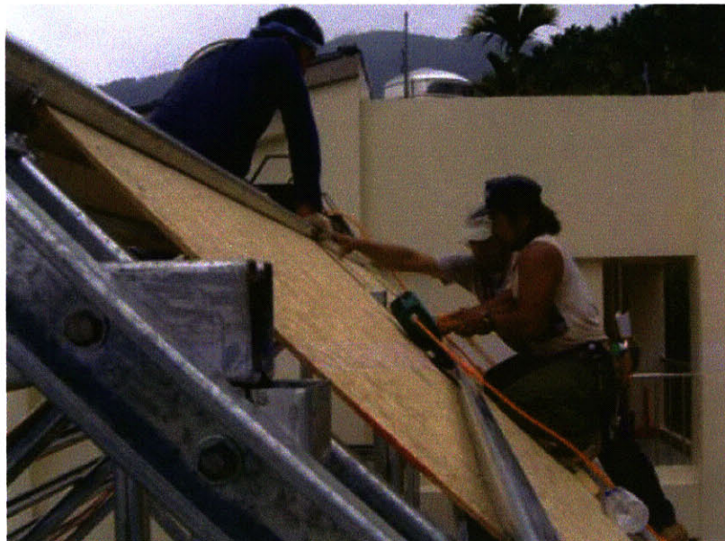
workers apply sheathing over a simple, bolted steel roof
