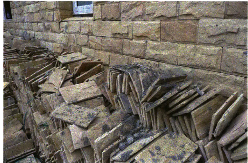
brick walls are clad with stone tile
