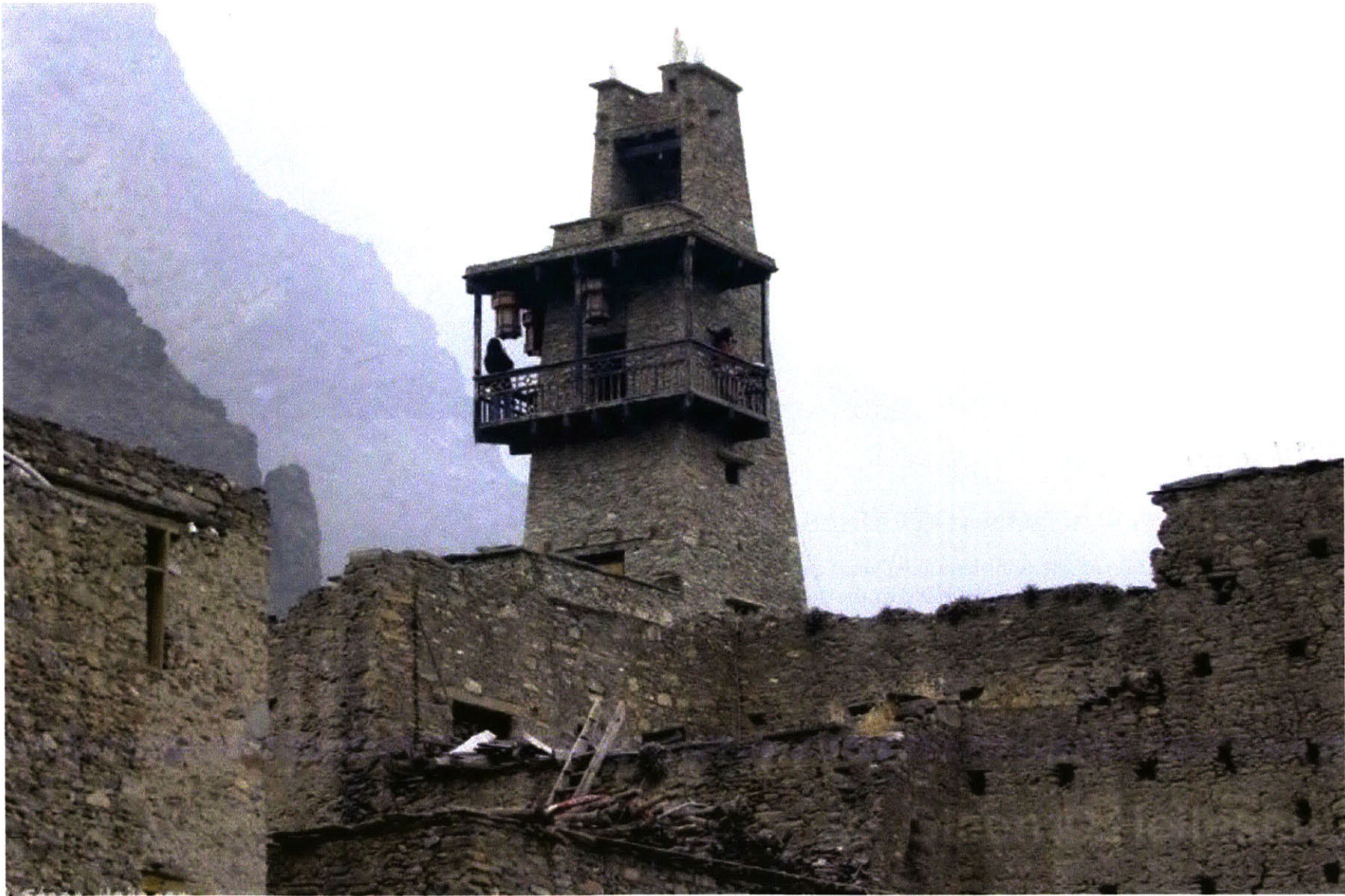
typical Qiang construction in Taoping Village with heavy, tapered walls, and attached wood balconies
