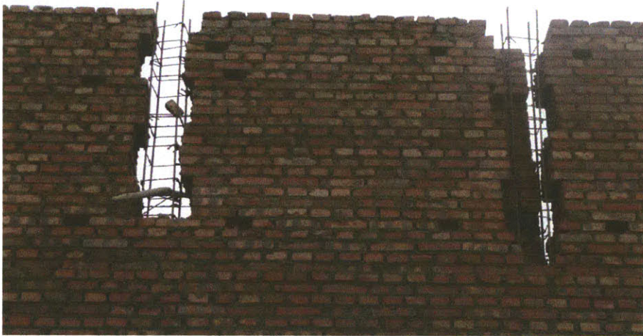
brick walls will be used as formwork for concrete columns
