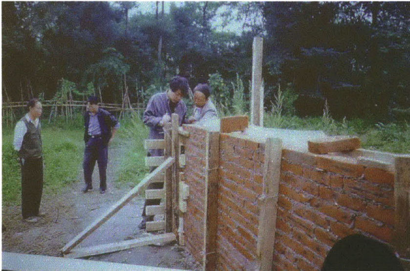
brick being used as formwork during construction of the Luyeyuan Museum
