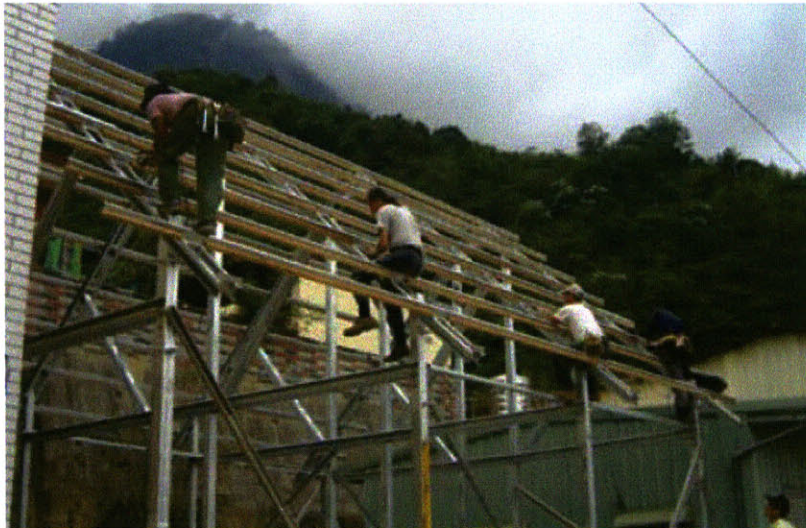
workers securing roof purlins
