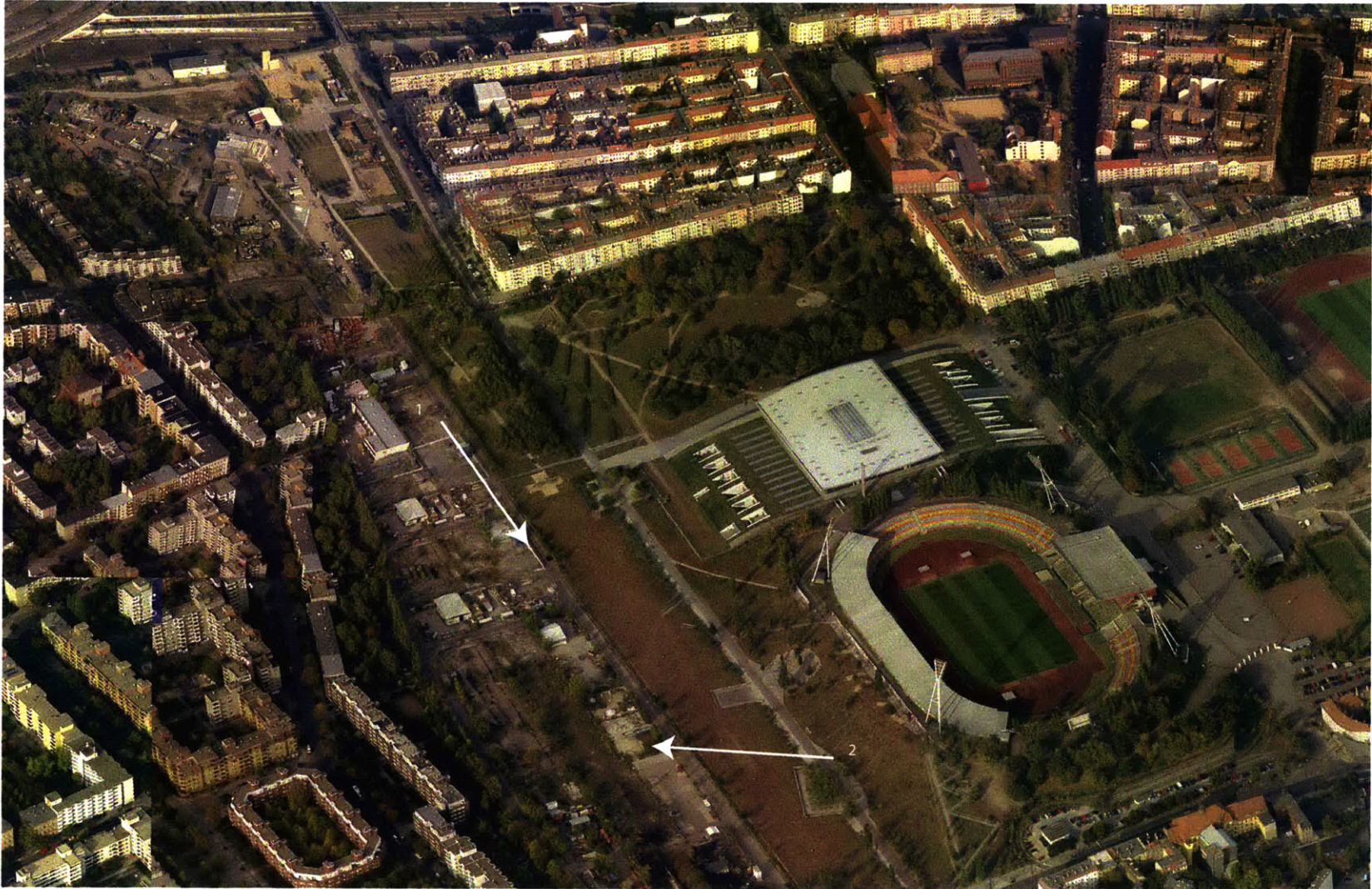
image source: http://www.googleearth.com Mauerpark Aerial Site Montage - Existing Conditions
