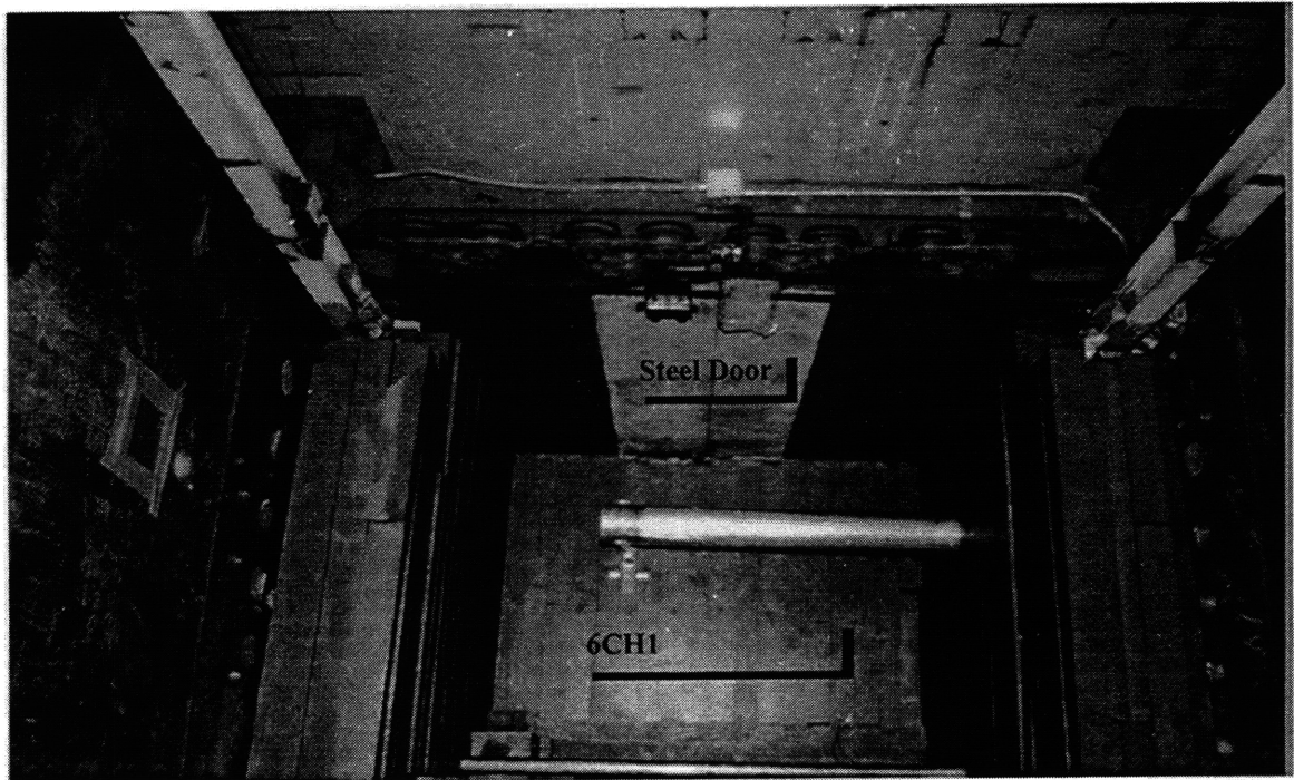
Figure 1.12: The hohlraum is viewed from above during renovation. The steel doors provide access to the thermal column. (Reactor Core is Toward Bottom of Page)
