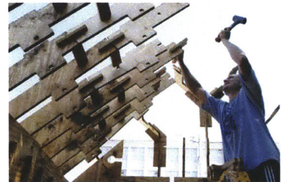
Construction underway; photograph illustrates component joints (image: http://ddf.mit.edu/projects/CABIN/cabin_full_plywood.html ).
