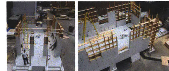
Construction in progress (image: http://www.momahomedelivery.org/ ).
