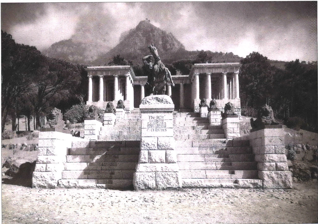
FIG. 4-40. RHODES’ MEMORIAL BUILDING.
