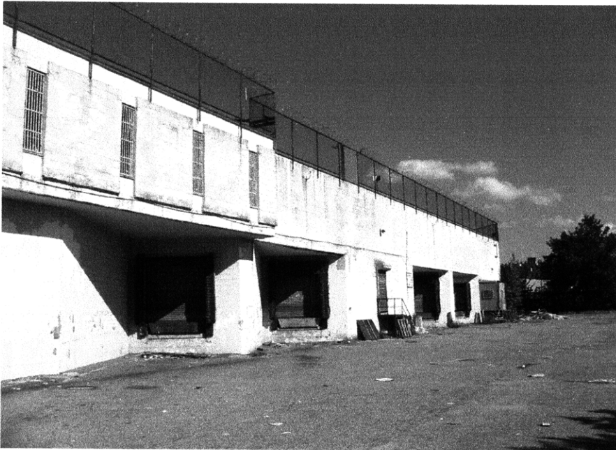
existing site c _ east facade
